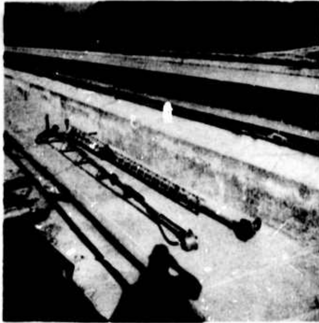
Figure 5-9 Belgian and Canadian Light Support Structures
