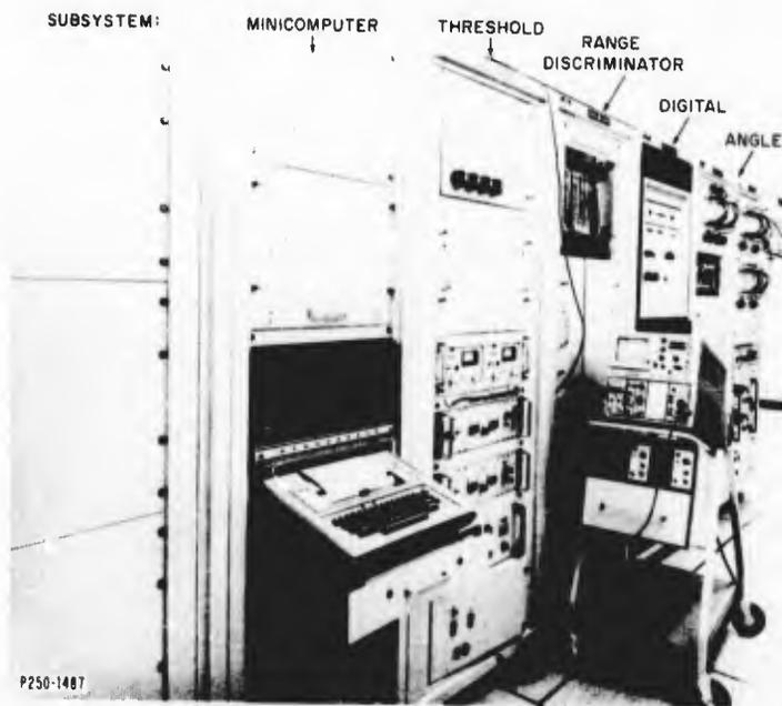
Fig. III-2. BATS SP equipment – front view.
