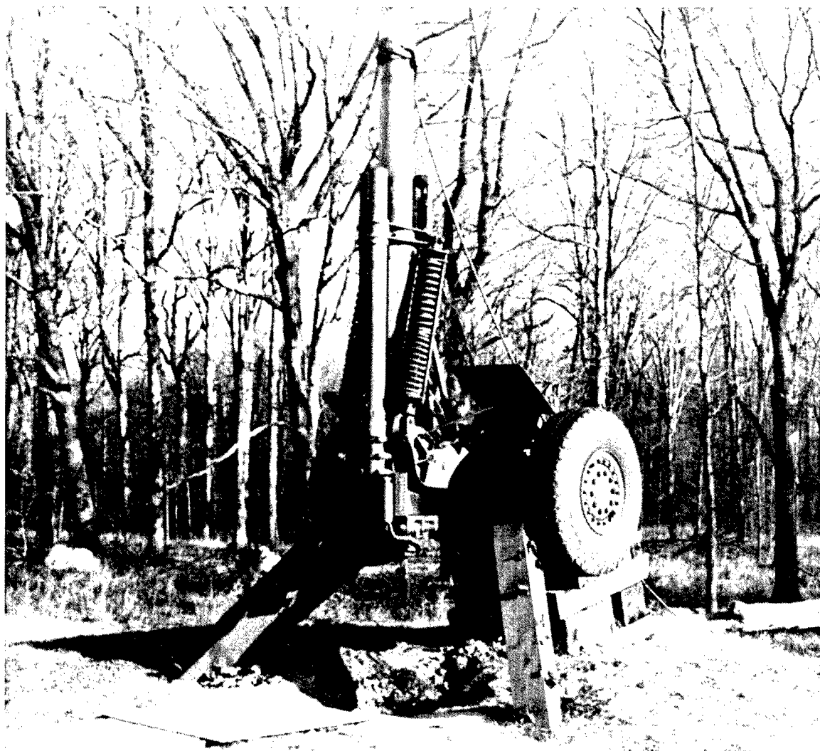
Figure 2. 155-mm Howitzer in Position for Vertical Firing.
