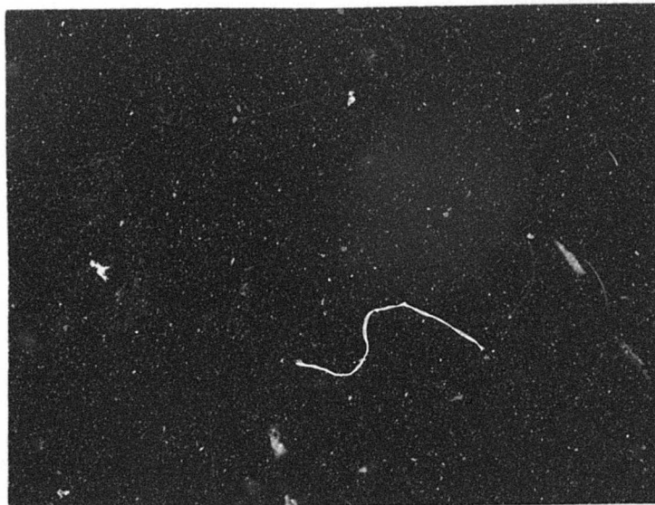
Figure 12. Close-up of cracking at doorway. (Crack was moistened prior to photographing to improve contrast.)
