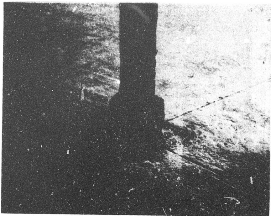
Figure 9. Functioning isolation joint of older construction, circa 1943.
