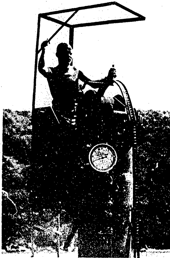
Fig. B51 - Tensionometer in use to control the descent of the launch barge
