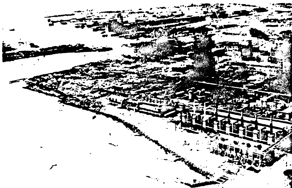
Figure B This illustrates all the significant explosion damage effects. The disaster caused by exploding ammonium nitrate on board two ships has been scaled at about 2.4 KT and involved a nearby chemical process plant, warehouses, grain elevator, refinery tankage, and many residences. Crater (water filled) at center left edge; massive diffraction loading damage
