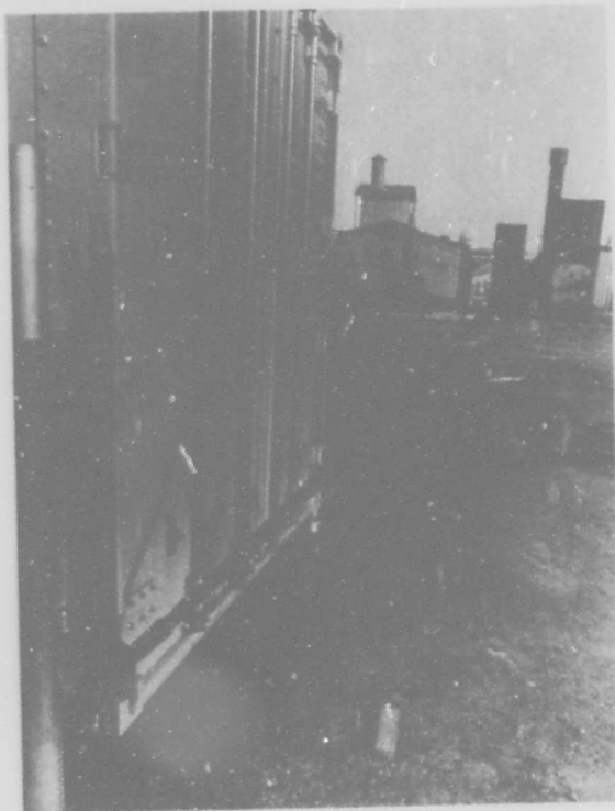
Figure 31. Exterior detail view of module showing support attached and jack in place.
