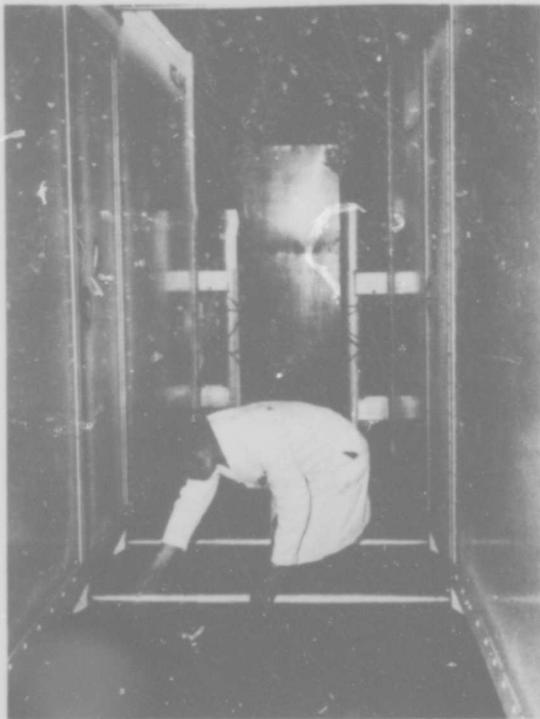
Figure 34. Telescoping supports for the flexible passageway.
