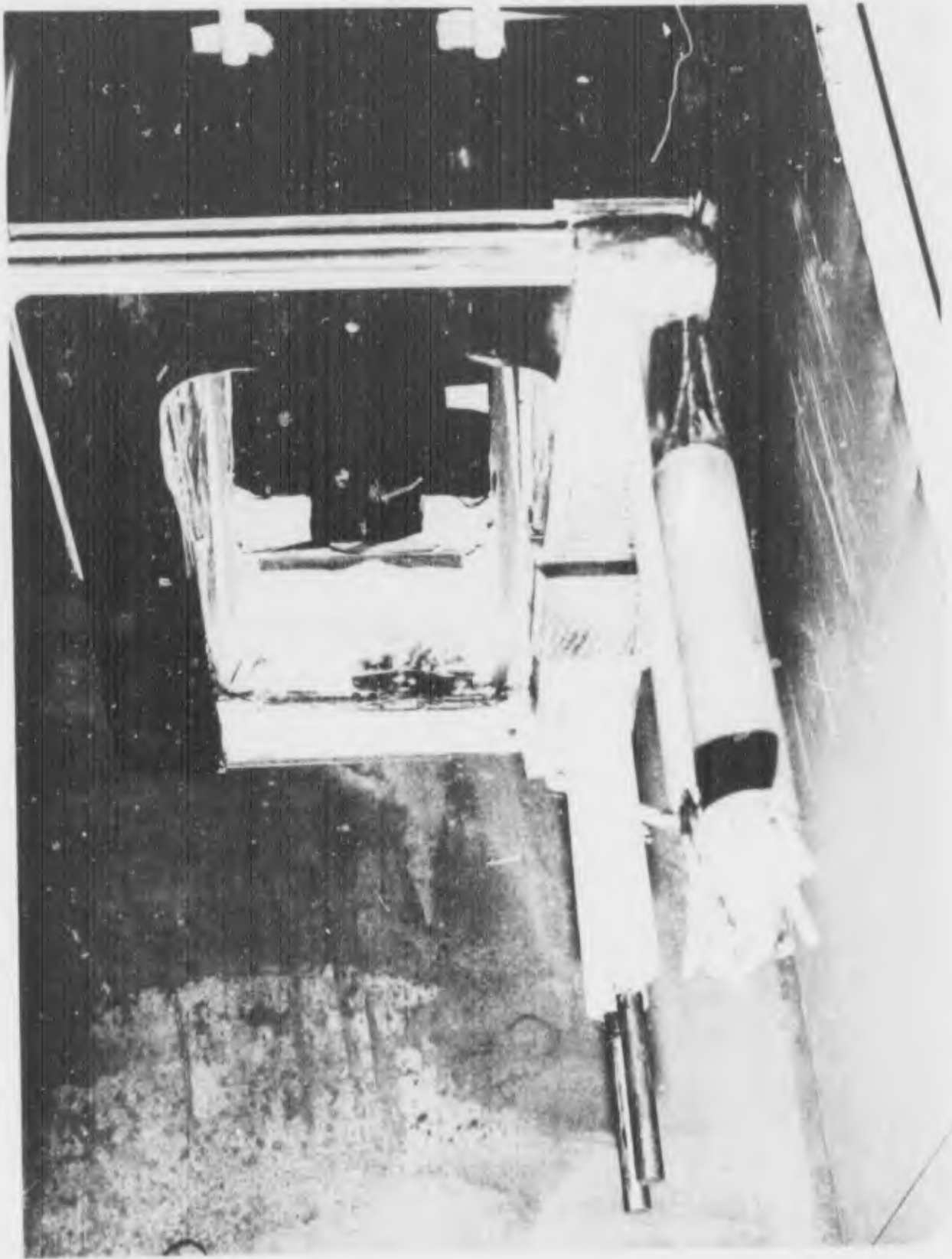
Figure 3. High Field End of the 4 Tesla Magnet. The Two Conductors at the Far End Were Repaired Last Year and the Second Failure Occurred at the Repaired Joint. The Failure Area is Visible to the Right of Leads.
