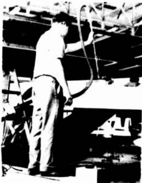
Figure 2. Wing Porosity Measuring Equipment.
