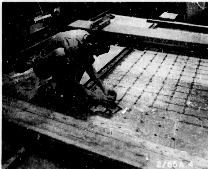
Figure 2. Coating of crack alarm grid wires with epoxy resin prior to concrete placement.
