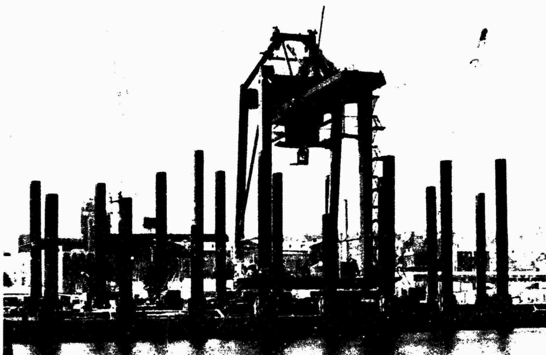
Fig. 71. DeLong barges supporting gantry cranes at Pier 13, Staten Island, New York
