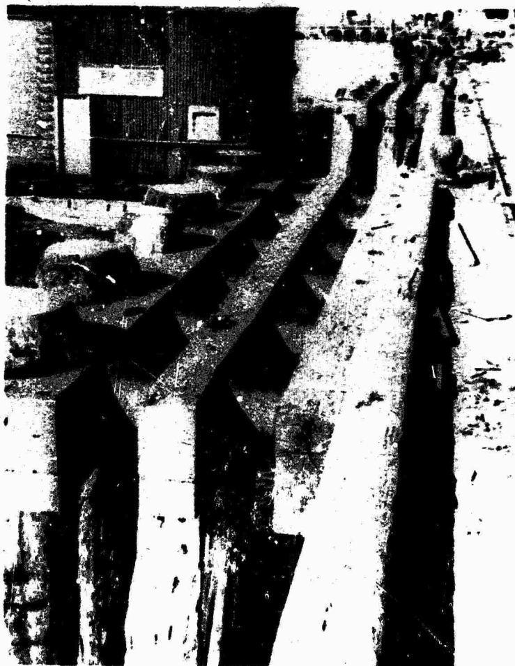
Fig. 90. Fendering example (cylindrical rubber fender in end compression)
