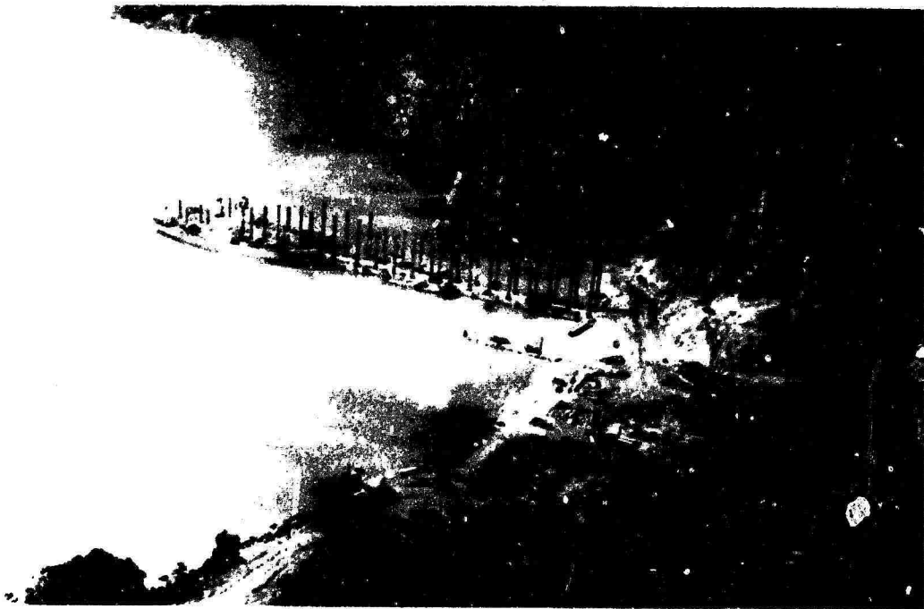
Fig. 69. Combination "A" and "B" barge pier and causeway at Vung Bo Bay, South Vietnam
