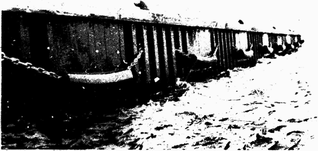
Fig. 88. Fendering example (draped cylindrical rubber fender)
