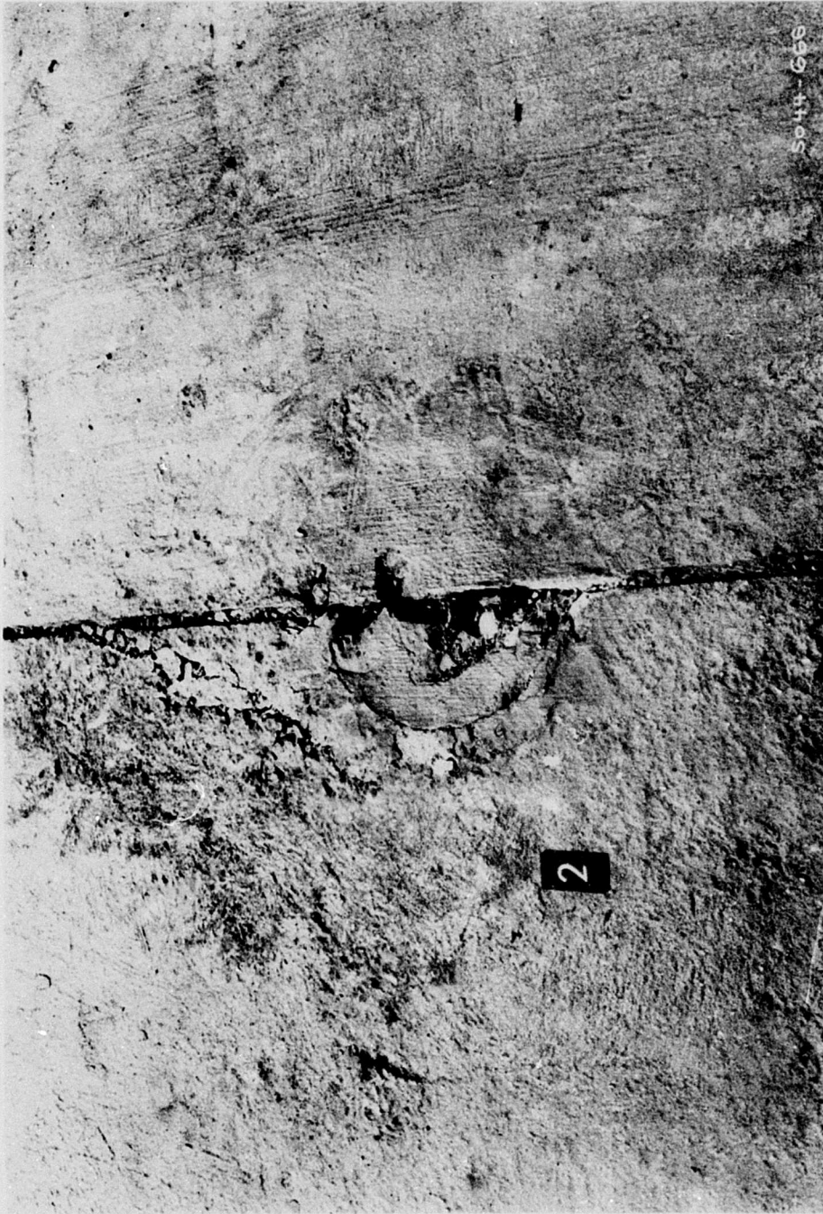
Figure 38. Flaking and spalling around the 8-in.-diam access holes filled with sand-cement grout (after 504 coverages).
