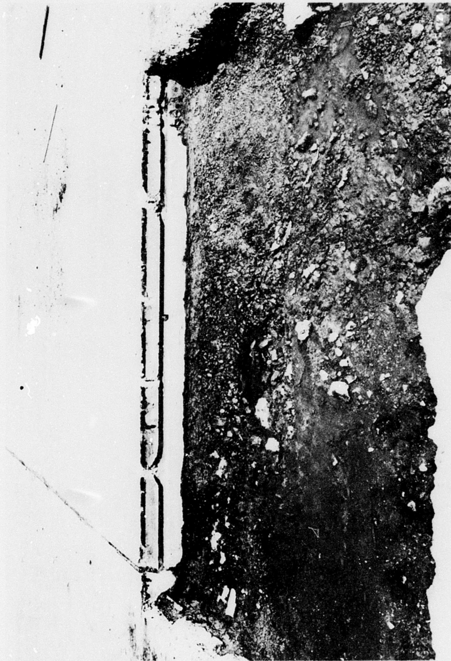
Figure 59. View of keyed longitudinal construction joint in item 4, 360-kip, 12-wheel-assembly lane after 6336 coverages.
