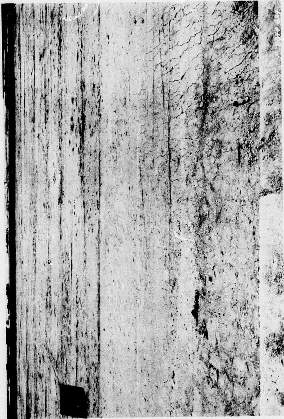
Figure 9. View of completed clayey gravelly sand base in item 1.
