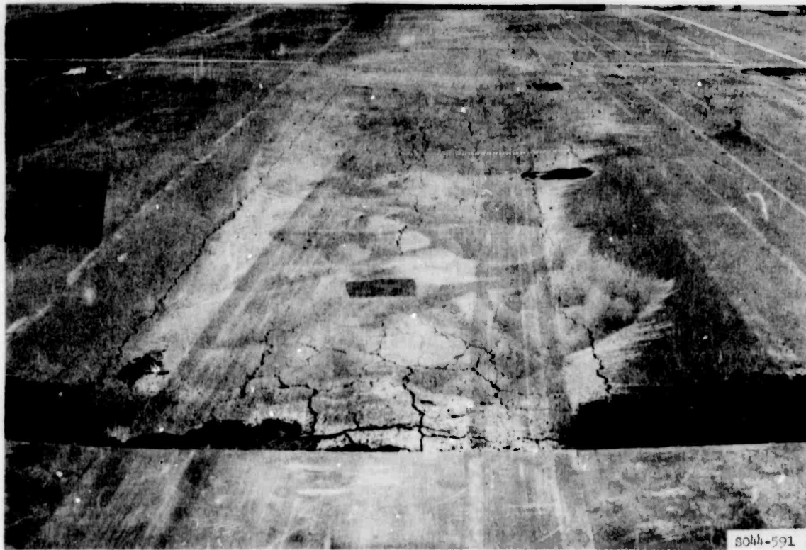
Photo B24. General view of item 3, lane 2, at failure (after 890 coverages of 200-kip, twin-tandem assembly)
