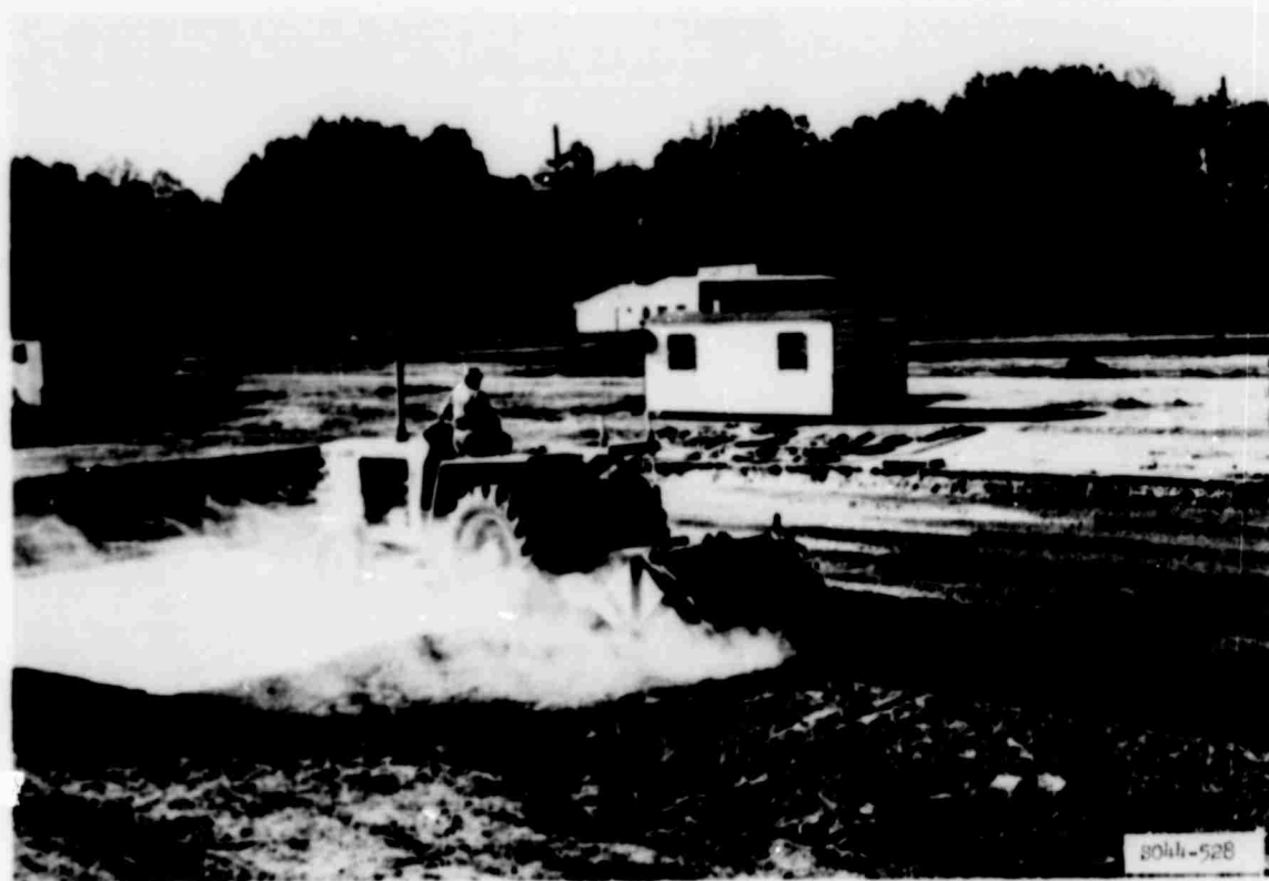
Photo 4. Mixing soil and stabilizing agent in items 1 and 2
