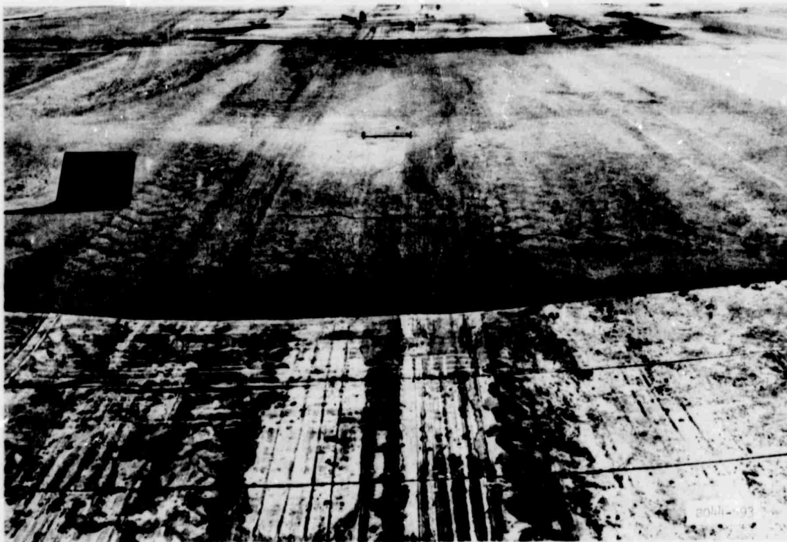
Photo B27. General view of item 4, lane 2, at failure (after 1810 coverages of 200-kip, twin-tandem assembly)
