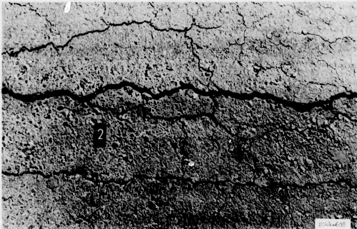
Photo B33. Close-up of severely cracked pavement in 100 percent coverage zone of item 2, lane 2, after 120 coverages of 50-kip, single-wheel assembly
