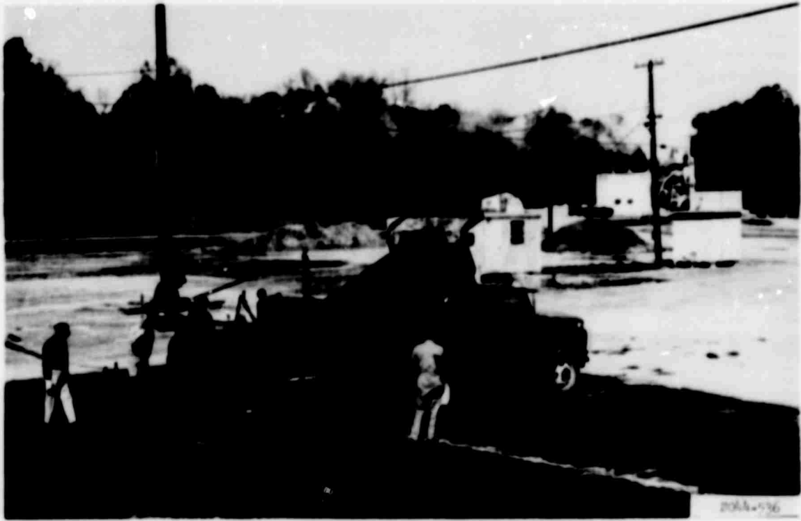
Photo 9. Placement of asphaltic concrete
