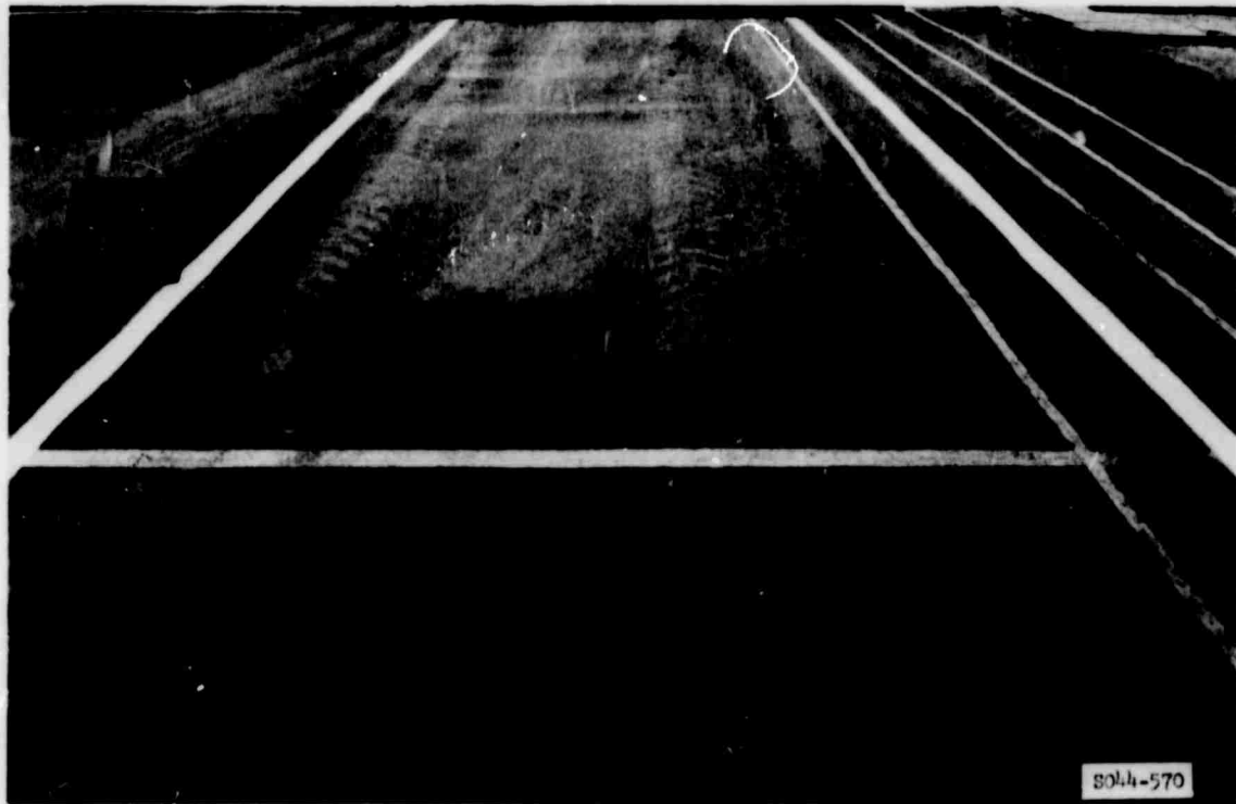
Photo B18. Item 2, lane 2, prior to traffic
