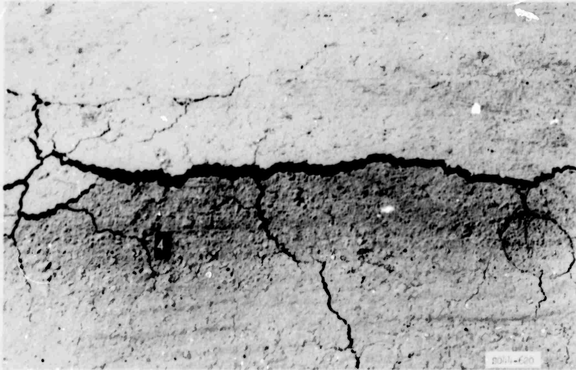
Photo B39. Severe cracking in the 100 percent coverage zone of item 4 at failure (after mixed traffic)
