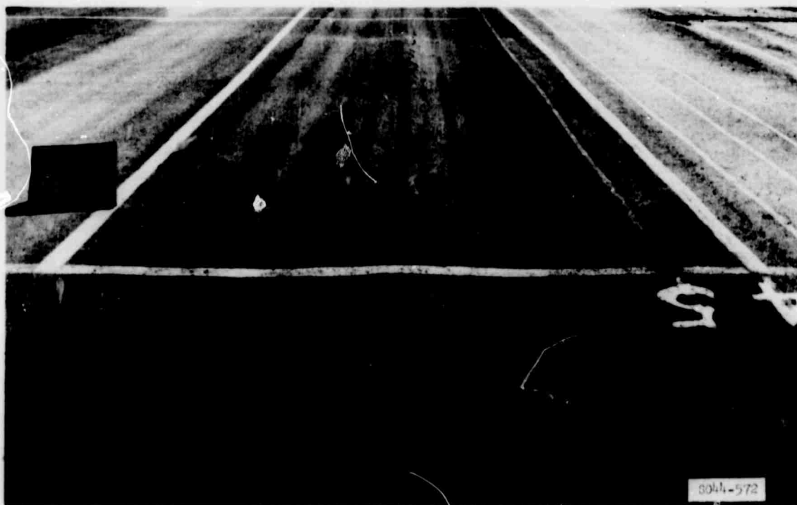
Photo B16. General view of item 1, lane 2, at failure (after 140 coverages of 160-kip, twin-tandem assembly)
