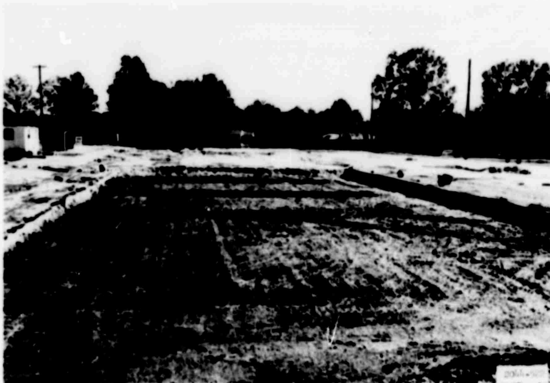
Photo 2. View of finished subgrade
