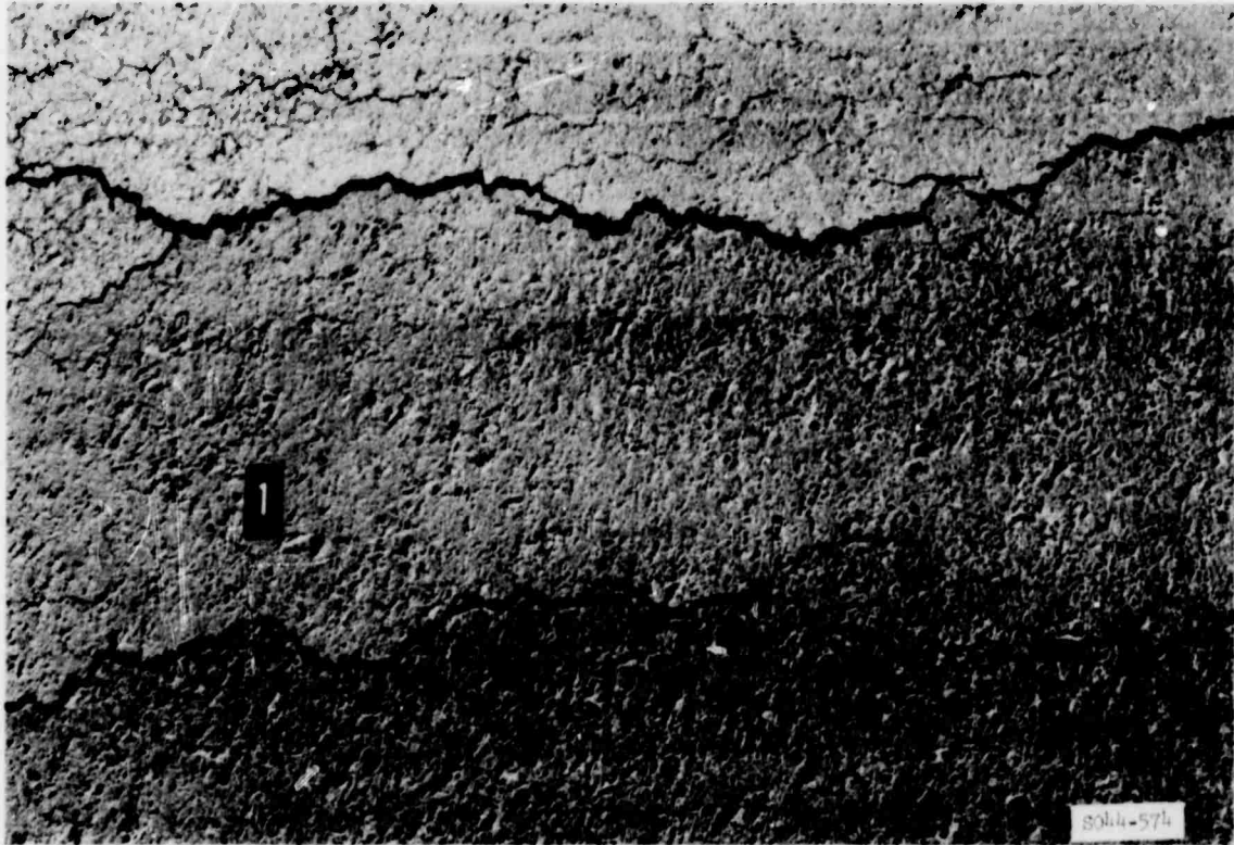
Photo B17. Close-up of cracks in 100 percent coverage zone in item 1, lane 2, at failure (after 140 coverages of 160-kip, twin-tandem assembly)
