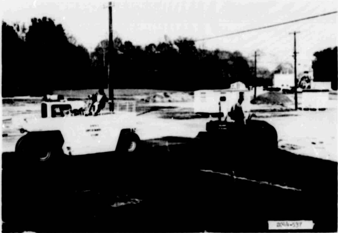
Photo 10. Breakdown rolling of asphaltic concrete with a steel-wheel roller and final compaction with a 30-ton rubber-tired roller
