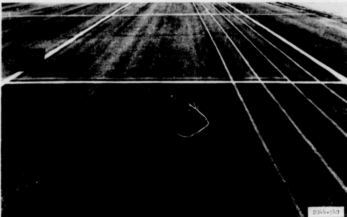
Photo B4. Item 2, lane 1, prior to traffic
