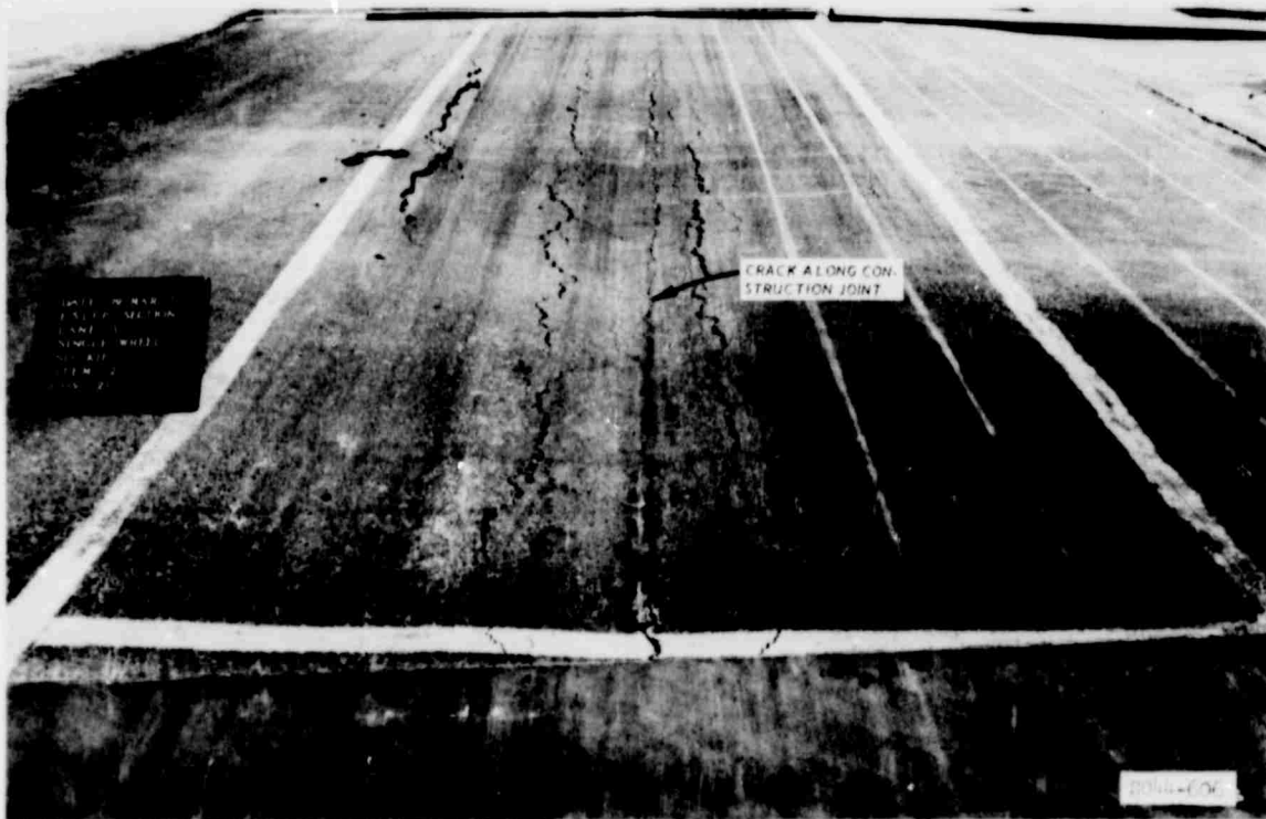
Photo B32. General view of item 2, lane 3, after 120 coverages of 50-kip, single-wheel assembly
