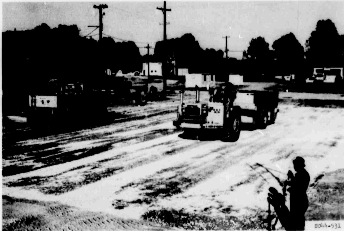
Photo 7. Compacting final lift of base course
