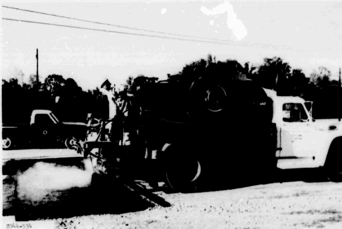
Photo 8. Priming crushed stone base course with MC-1 cutback asphalt
