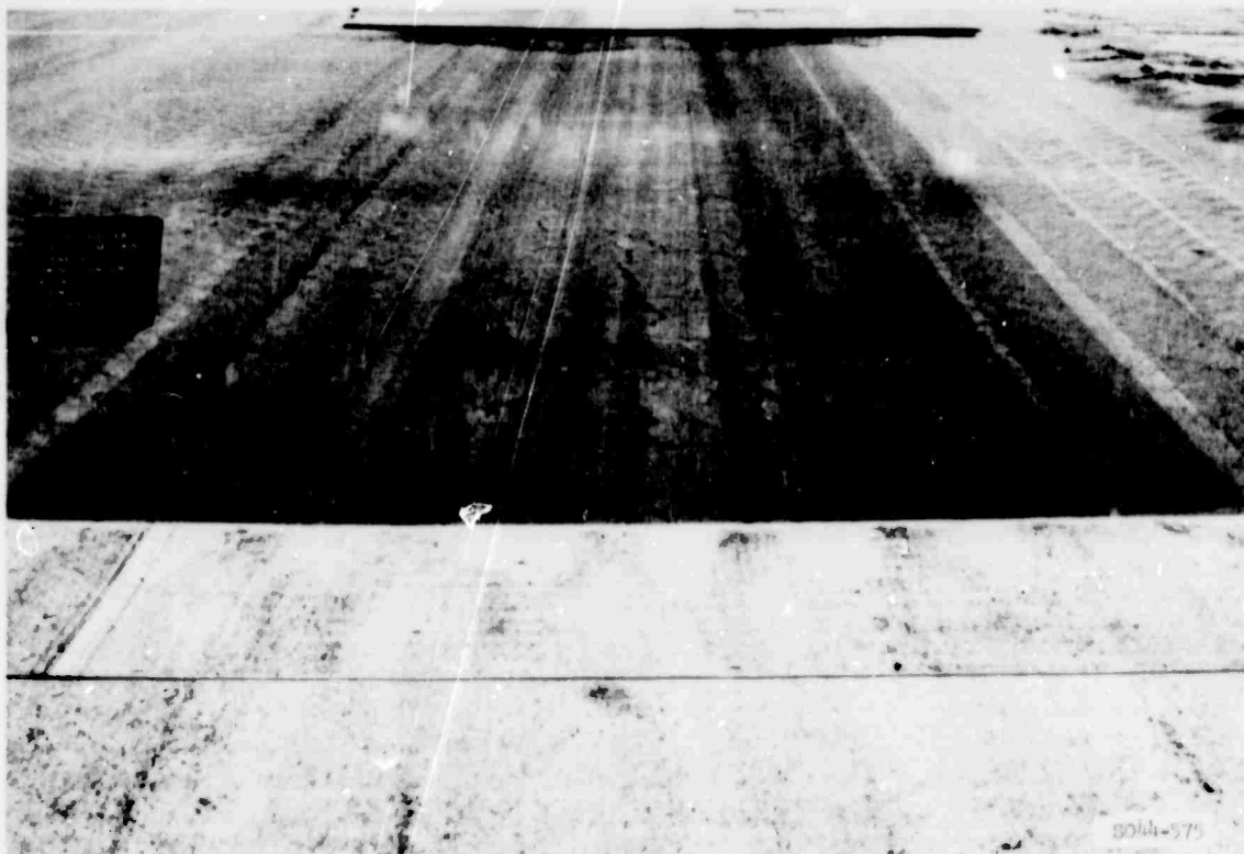
Photo B20. General view of item 2, lane 2, at failure (after 1000 coverages of 160-kip, twin-tandem assembly)
