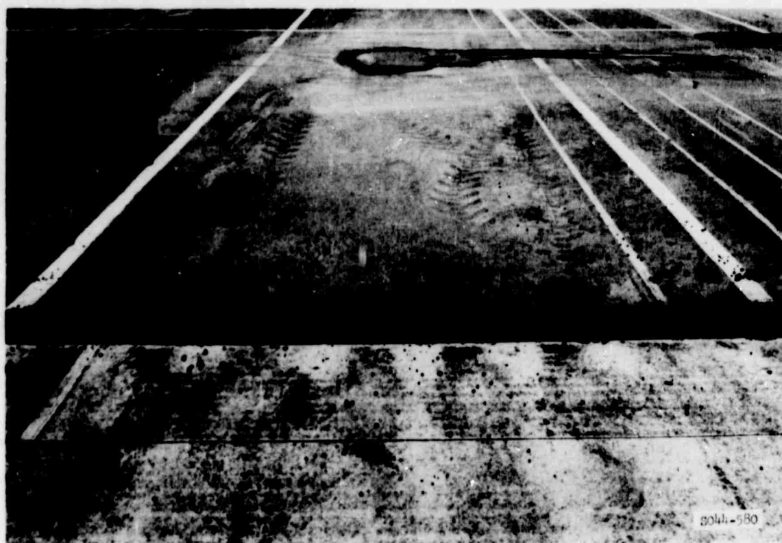
Photo B22. Item 3, lane 2, prior to traffic
