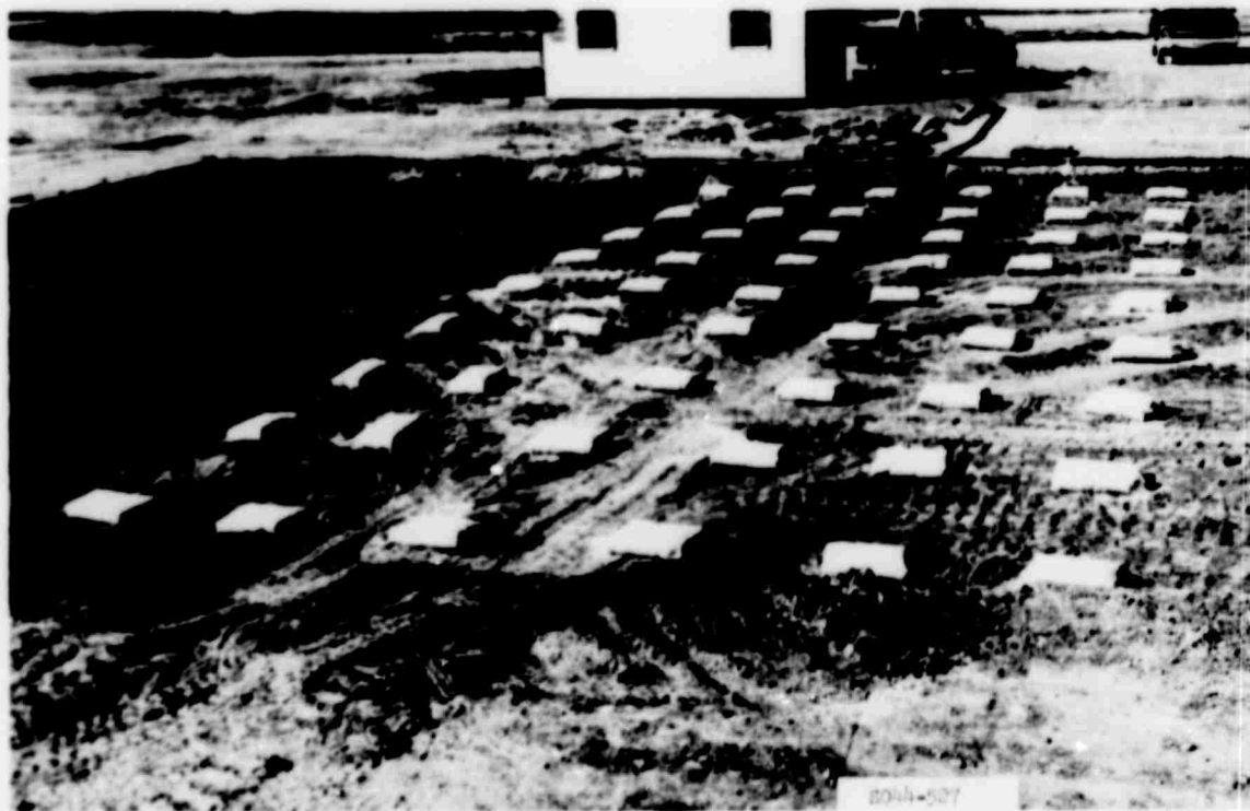
Photo 3. Bags of stabilizing agent placed at predetermined intervals for desired percent of treatment
