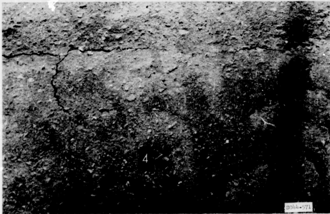
Photo B14. Small cracks extending from construction-joint crack in item 4, lane 1, after 10,406 coverages of 360-kip, 12-wheel assembly
