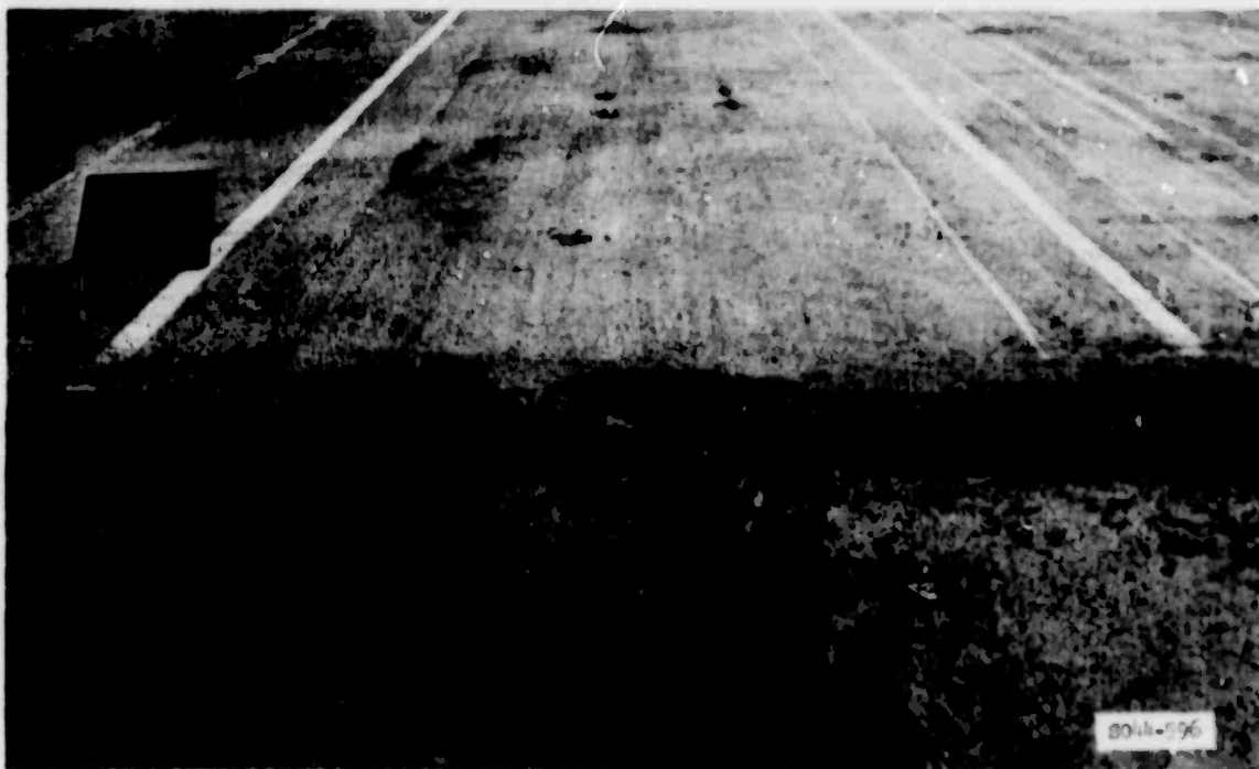
Photo B38. General view of item 4, lane 1, after 10,406 coverages of the 360-kip, 12-wheel assembly and prior to trafficking with the 75-kip, single-wheel assembly
