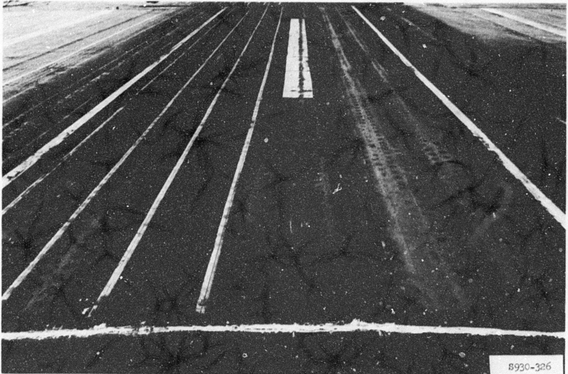
Photo 69. Condition of membrane sheet 1 of test section 1 after 910 coverages
