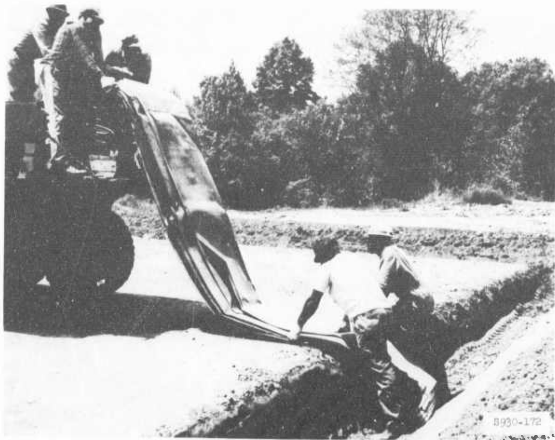
Photo 29. Placing membrane end in anchor ditch
