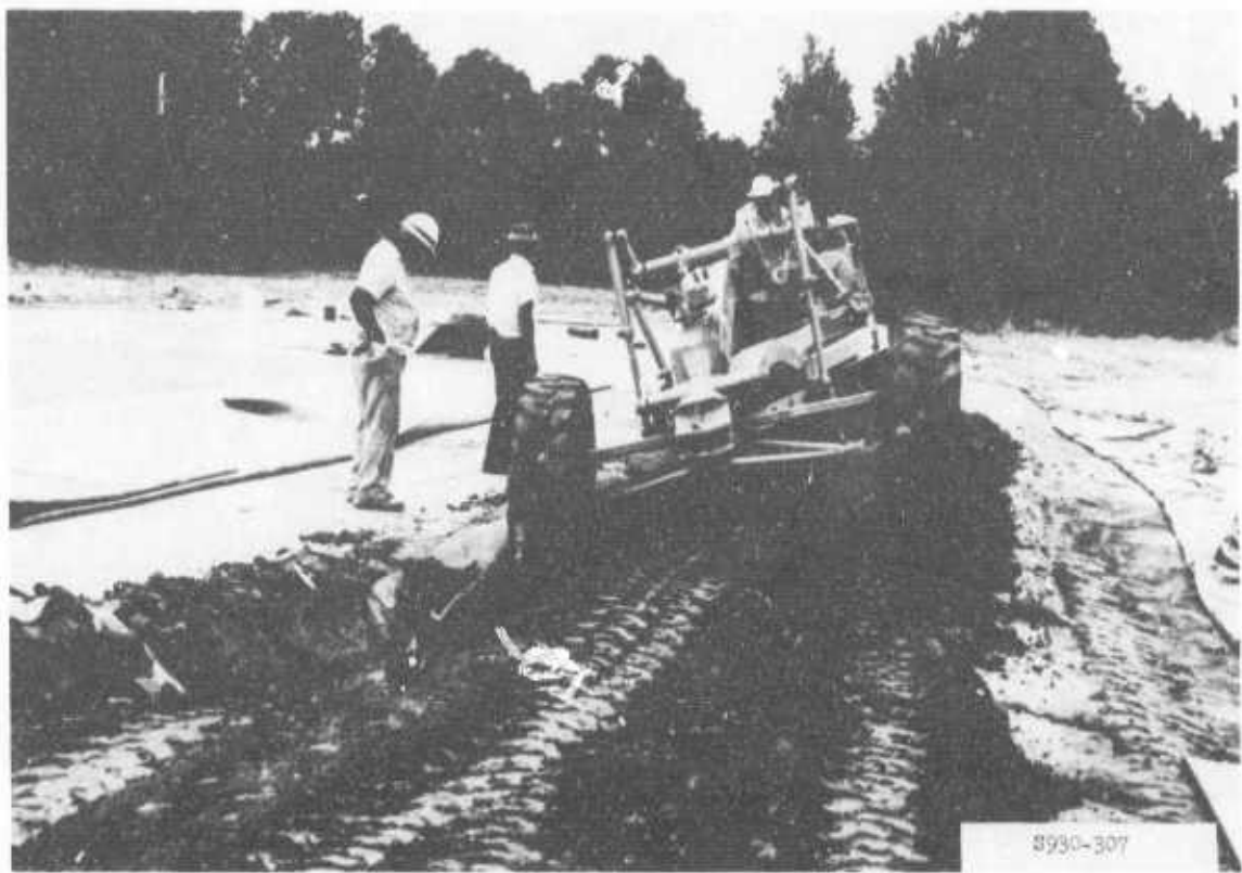
Photo 57. Motor grader removing remainder of sheet 3, test section 1, that was buried in anchor ditches
