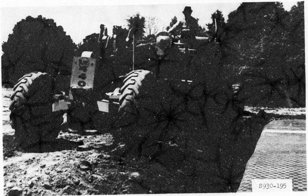
Photo 34. Motor grader backfilling anchor ditch
