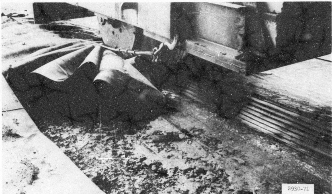
Photo 17. Failure of run 1 of XW18 membrane section 1 after ten repetitive skids
