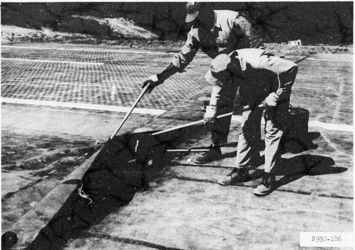
Photo 36. Overlapped end of second sheet raised with 48-in.-long paint roller handles while applying adhesive to joint
