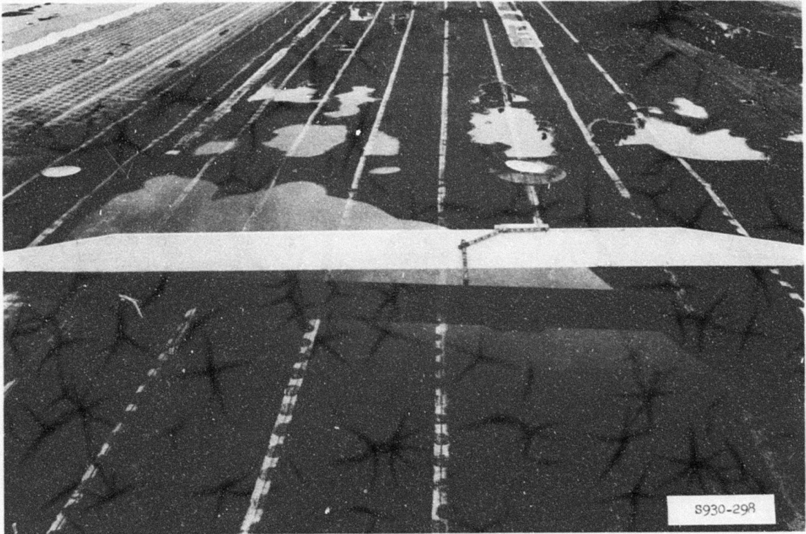
Photo 55. Rutting of subgrade of test section 1, sta 1+05, after 538 coverages
