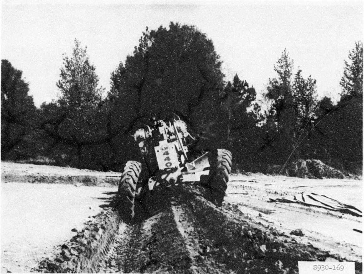
Photo 28. Motor grader constructing 2-ft-deep anchor ditch prior to placement of membrane sheets
