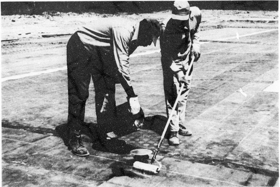
Photo 38. Applying adhesive to gasket of anchor at joint between second and third sheets
