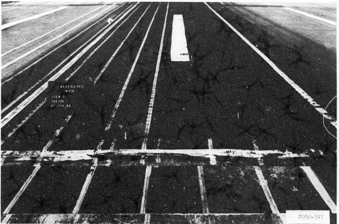
Photo 66. Sheet 3A of test section 1 after 200 coverages (total of 738 coverages on test section)
