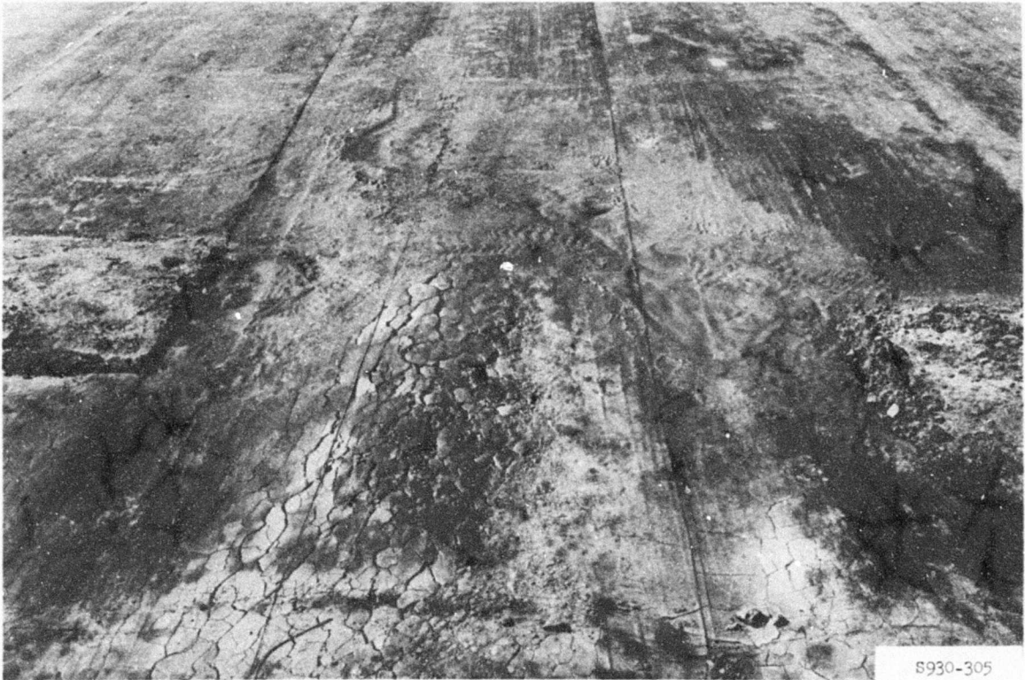
Photo 59. Condition of lean clay subgrade of test section 1, sta 1+05, after 538 coverages
