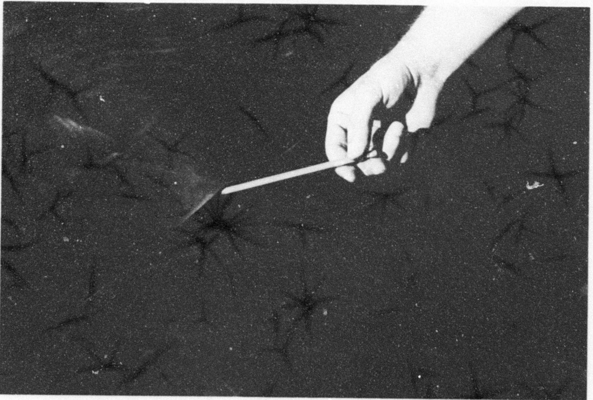
Photo 47. Edge of 3-ft-wide reinforcing strip on adhesive construction joint worked loose by test wheel (100 coverages on test section 1)
