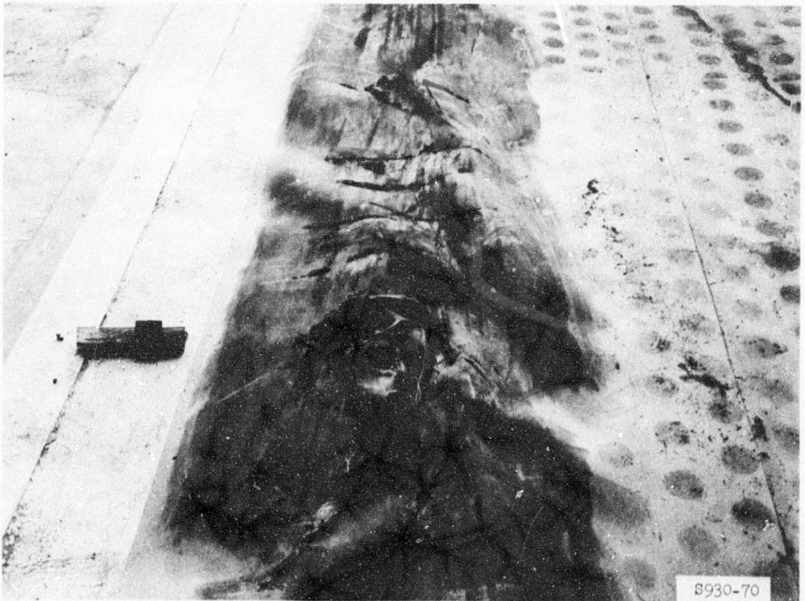
Photo 16. Extensive top-ply failures after sixth repetitive skid on run 1 of XW18 membrane section 1
