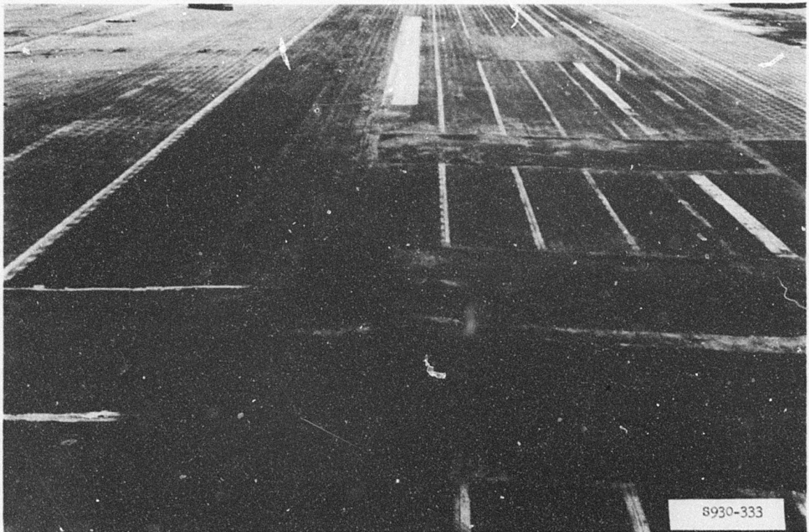
Photo 73. Condition of sheet 2 of test section 1 after 1200 coverages
