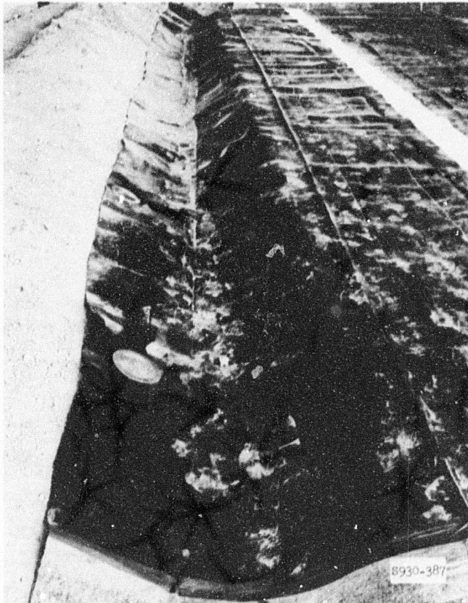
Photo 42. Steel anchors driven through surfacing on outside slope of ditch
