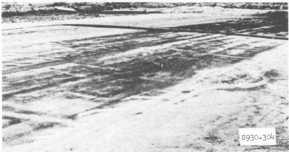
Photo 58. Sheet 2 of test section 1 cut along sides and folded back for repair of subgrade (538 coverages); note depressed area at center
