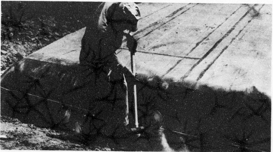
Photo 32. Driving steel anchor through membrane placed in anchor ditch
