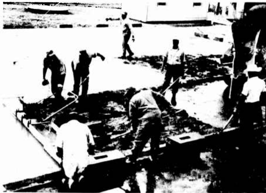
Figure 5. Vibrating screed.
