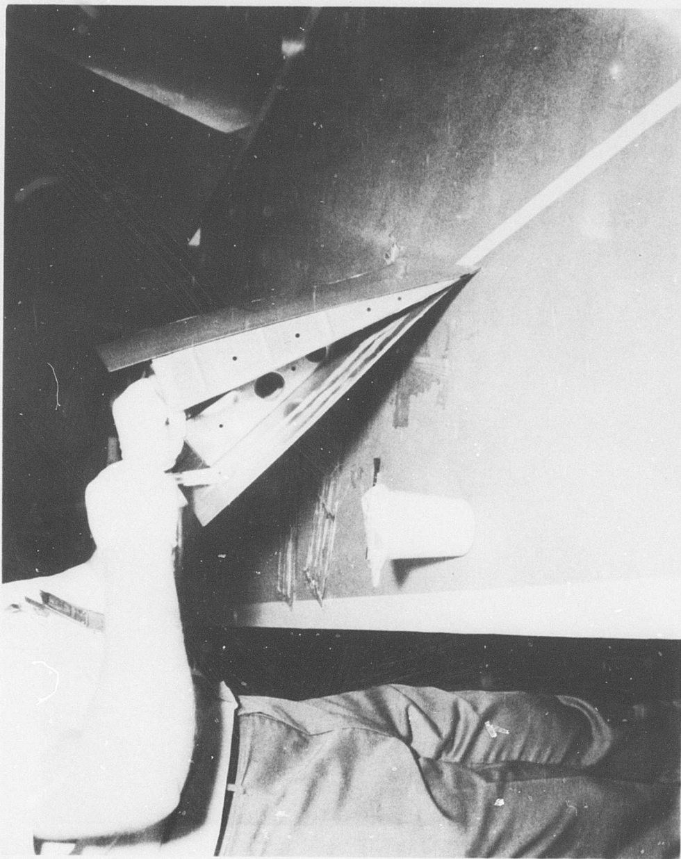
Figure 56. Application of Mixed Selected Adhesive to Universal Pocket.
