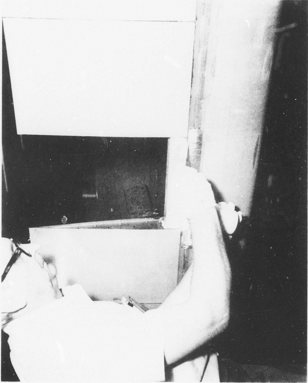
Figure 37. Applying Candidate Adhesive to Spar.
