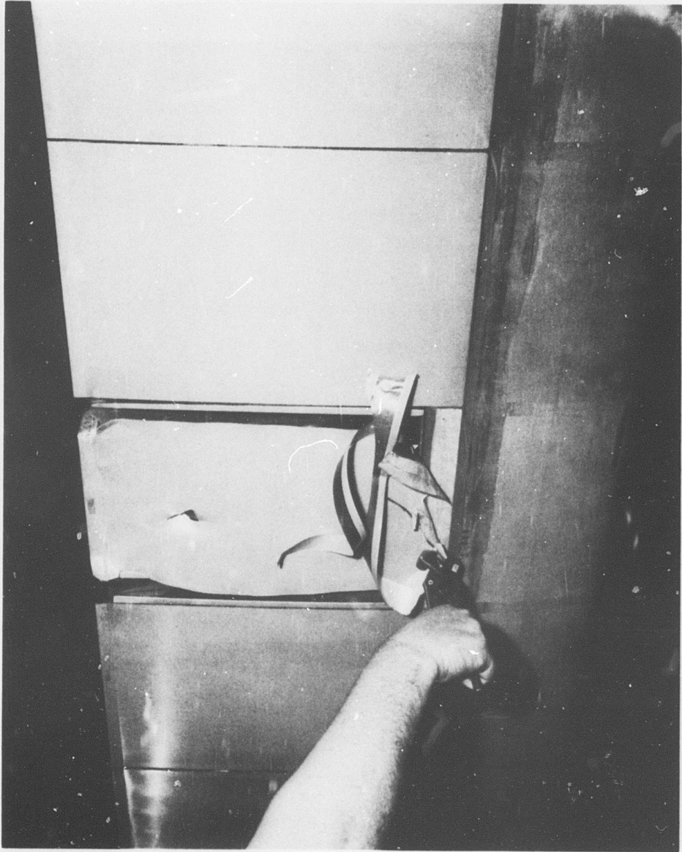
Figure 50. Removing a Damaged Blade Pocket.
