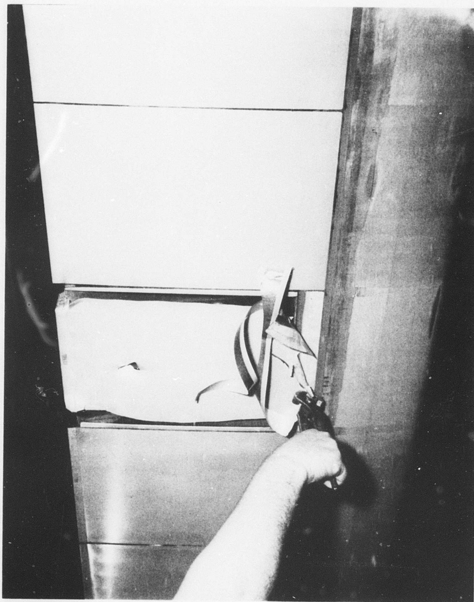
Figure 32. Removing a Damaged Pocket.
