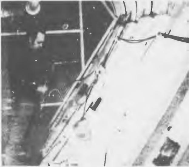
Wiring Hull Strain Gages
