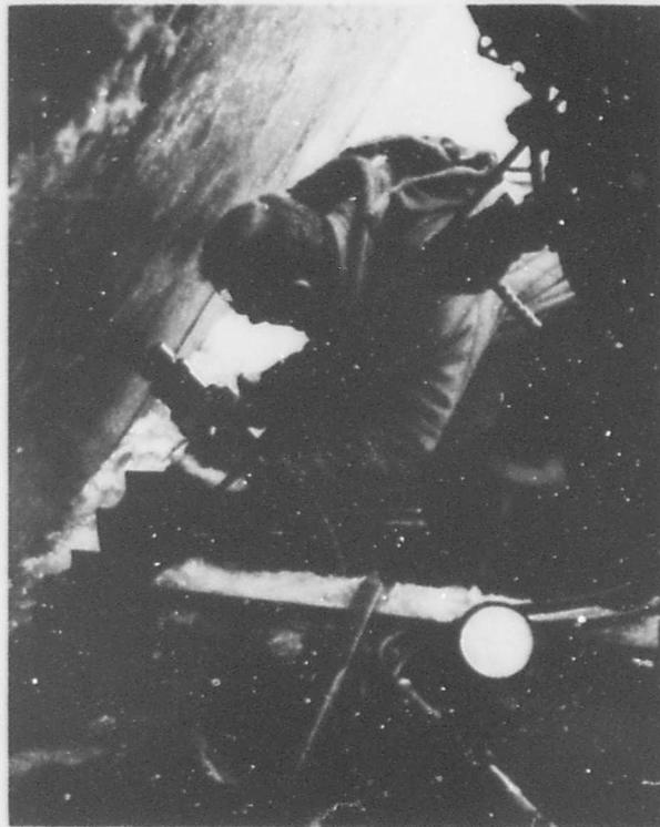
Adjusting Hydraulic Jack Against the Hull
