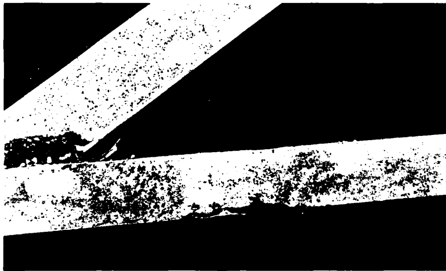
Figure 7. Pitting on base ring brace.
