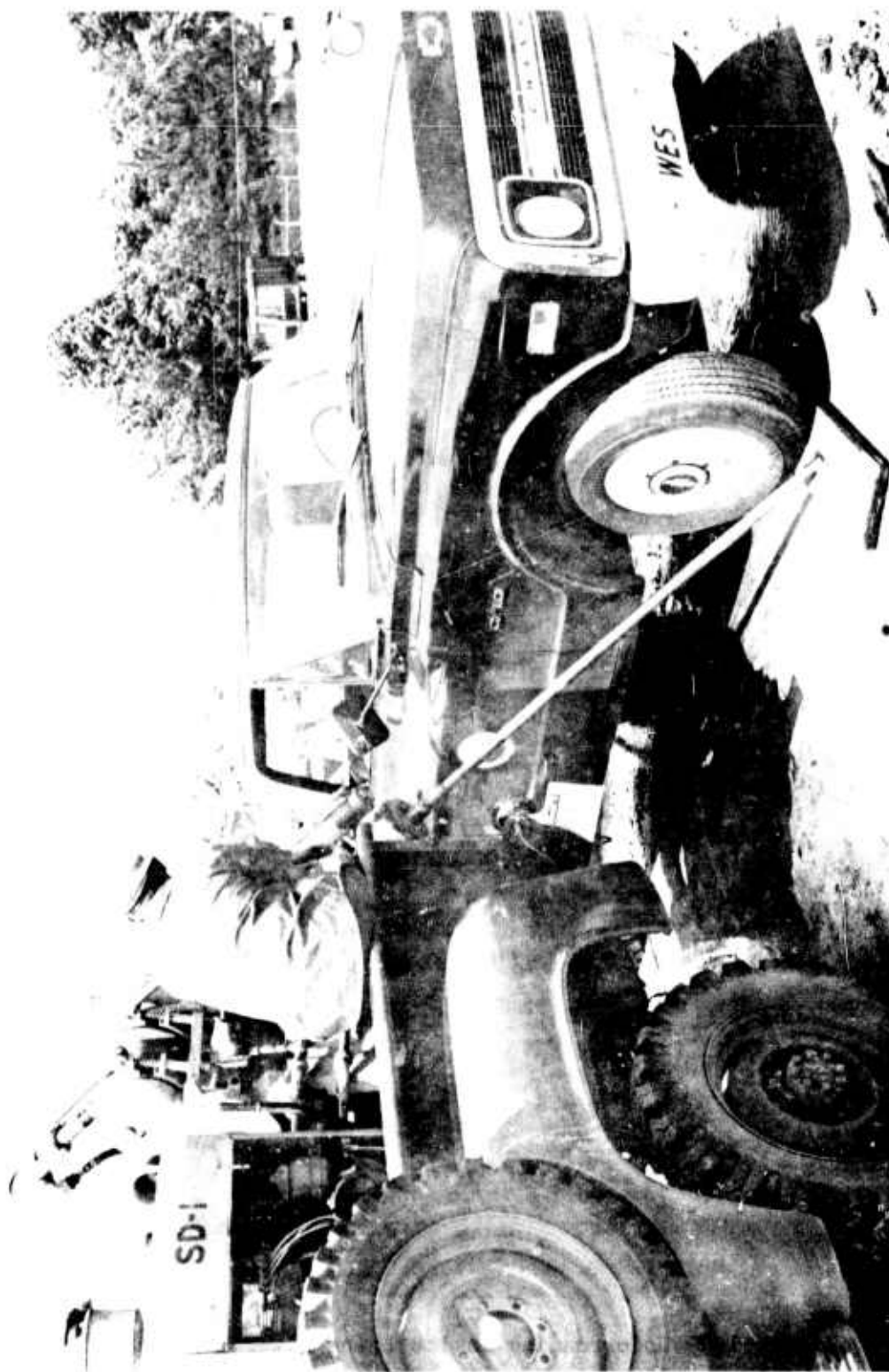
Figure 18. Coring 1-1/2-in.-diam hole at a 45° angle through the longitudinal joint in item 2.
