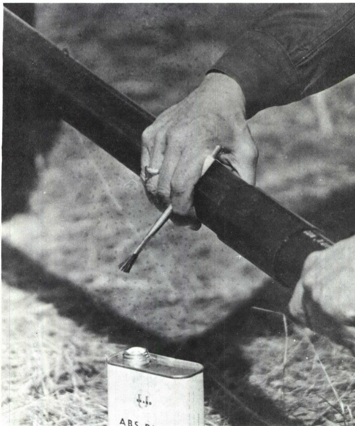
FIGURE 8. Assemble rest of 2" pipe - adhesive is applied to pipe end then coupling end of next piece of pipe is slid on. Do this fast - adhesive sets up rapidly.
