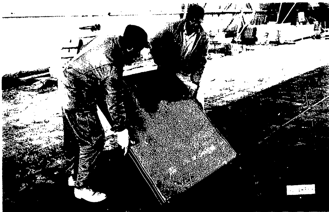
Fig. 4. Interlocking female connector with male connectors during assembly of MX19 panels
