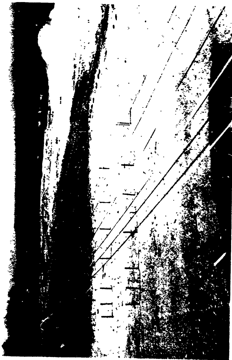
Fig. 4. Installation of main cables between berms.
