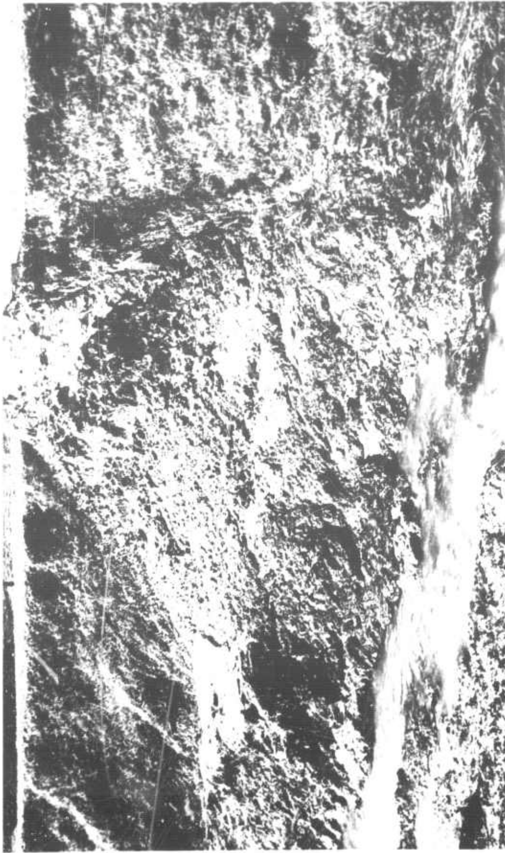
Photograph 35. Laminated dike in creek after attack by overflow current. Note disappearance of asphalt apron across creek channel
