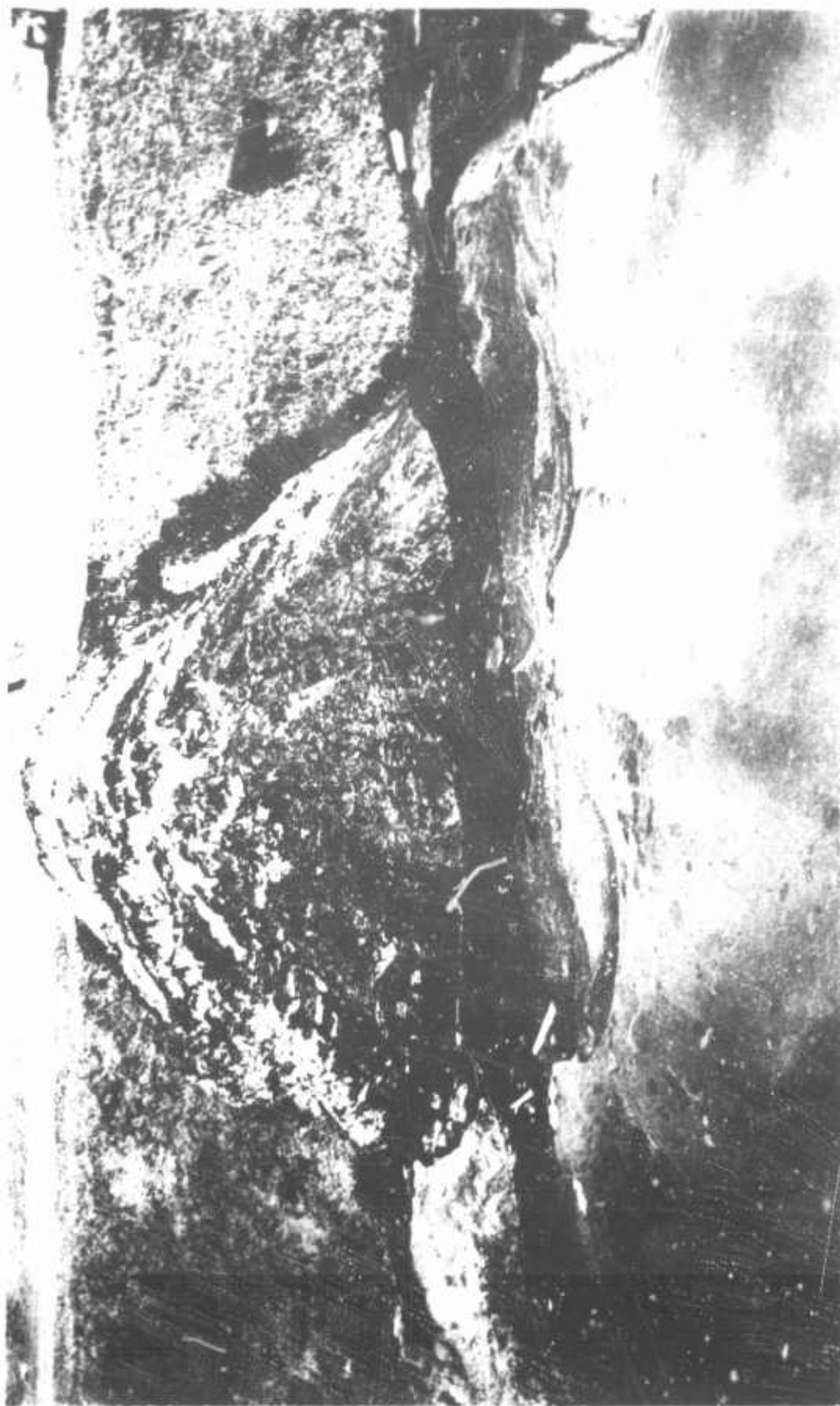
Photograph 32. Completed laminated dike in creek 12 hours after placement. Note sloughing and broken seal at top. Asphalt on the water floated during placement
