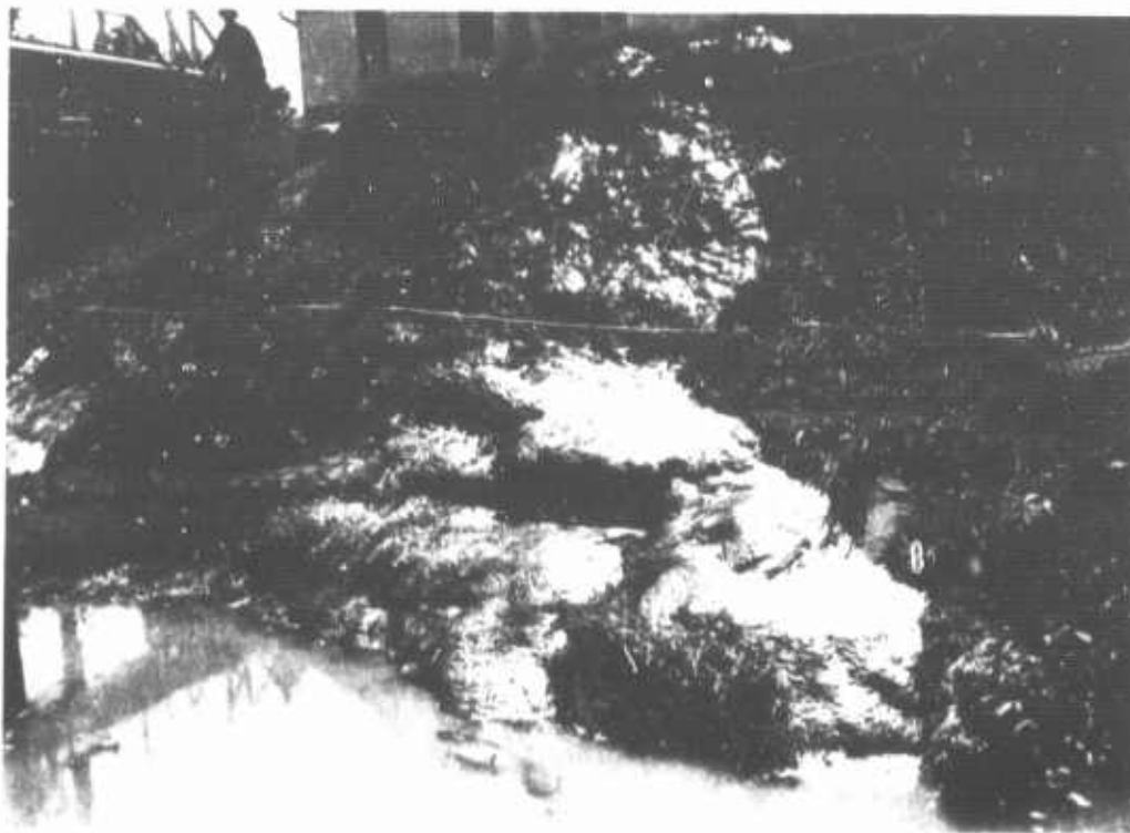
Photograph 22. Close-up of 30 per cent mix noted in photograph 20 shortly after placement. String line indicates water elevation during placement
