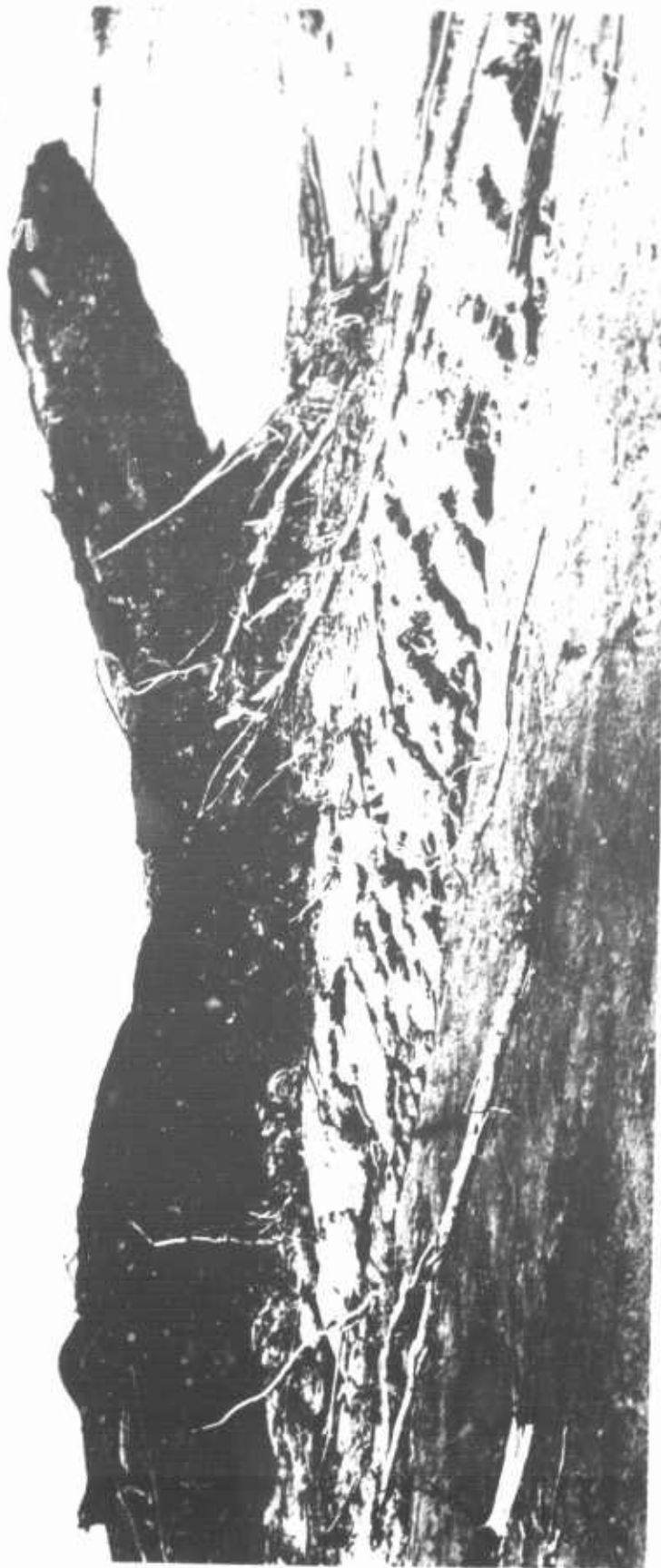
Photograph 36. Low-water view of asphalt dike or groin placed near the lower end of existing revetment at Fittler Bend, Mississippi River. Dike was constructed during high water.
