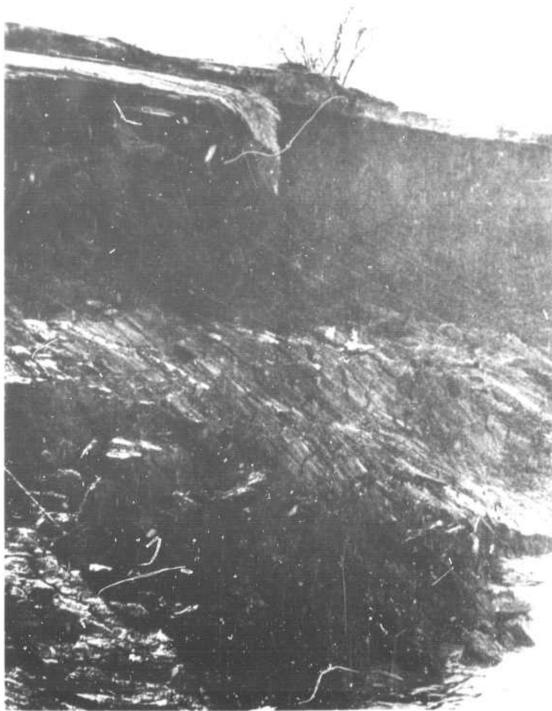
Photograph 41. Close-up of failed area at upstream end of False Point revetment in 1950
