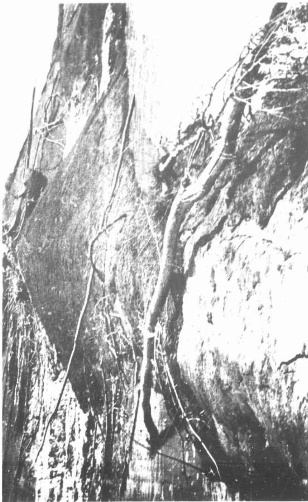
Photograph 37. Close-up of lower tier of Fittler dike. Note displaced seal coat and cracks in core
