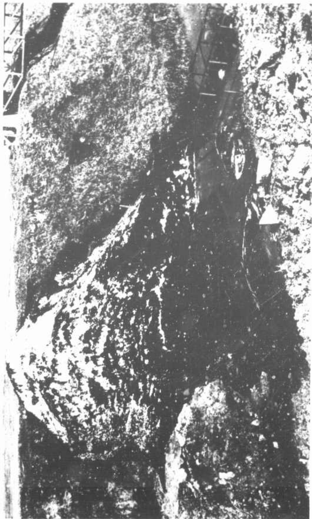
Photograph 34. Condition of laminated dike after exposure to sunbaking for five days. Note asphalt apron across channel, partly exposed
