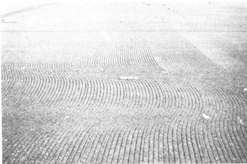
Figure 25. Washington National Airport -- Shifting of pavement surface in area of north end of runway.
