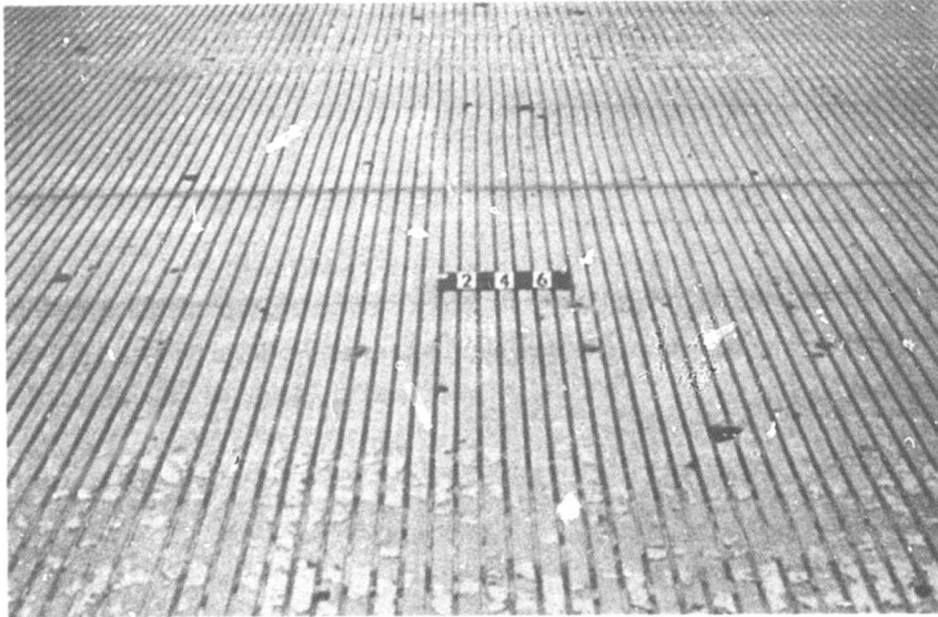
Figure 3. Kansas City Municipal Airport -- PCC grooving (small holes in surface are weatherouts).
