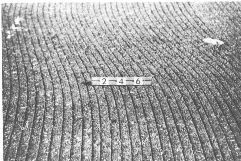
Figure 26. Washington National Airport -- Closeup showing distortion of grooves - same area as Figure 25.
