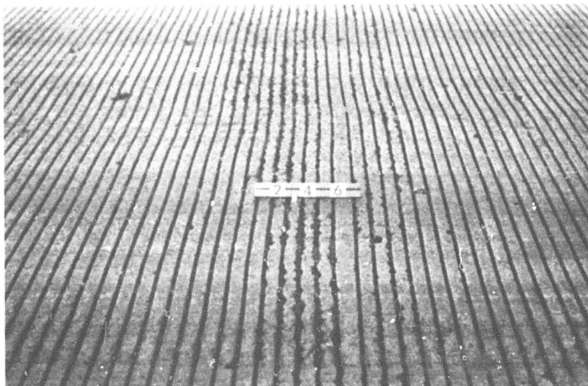
Figure 2. Kansas City Municipal Airport -- Deterioration of AC grooving located near runway end (36)
