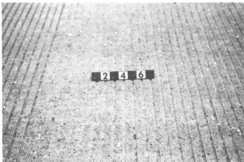
Figure 32. Beale Air Force Base -- Typical grooving in Runway 14/32.
