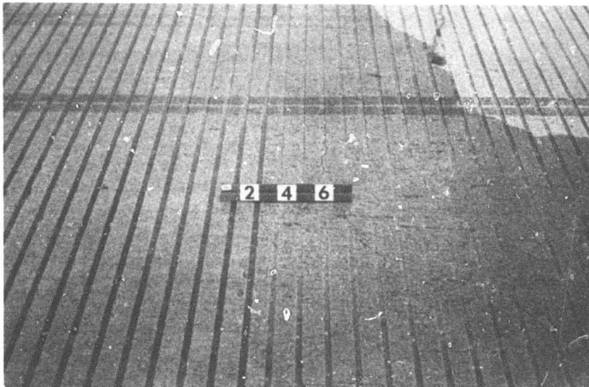
Figure 10. Chicago Midway Airport -- Deficiency in grooving due to low area in pavement surface.
