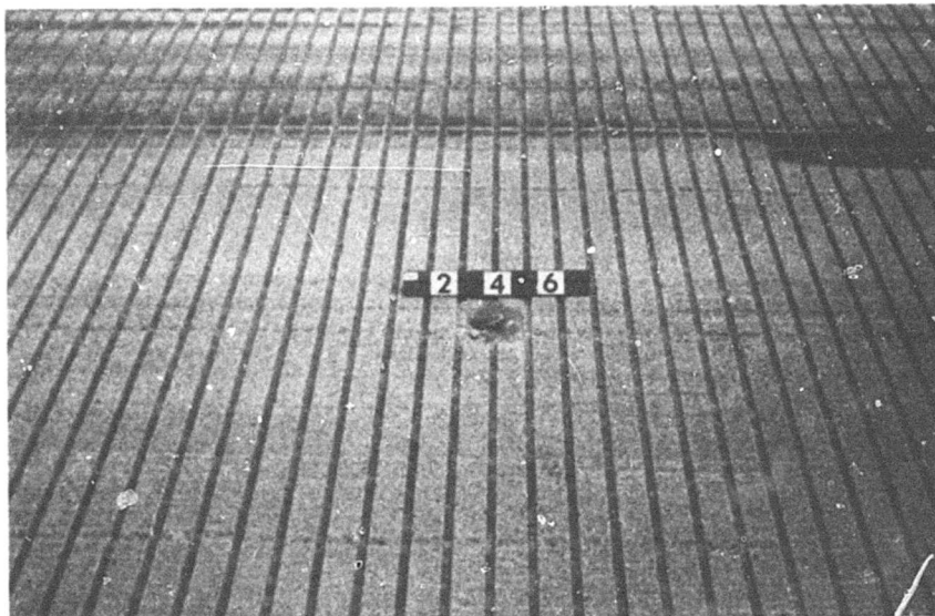
Figure 12. Chicago Midway Airport -- Close view of a weatherout, 1500 feet from northwest end of runway.
