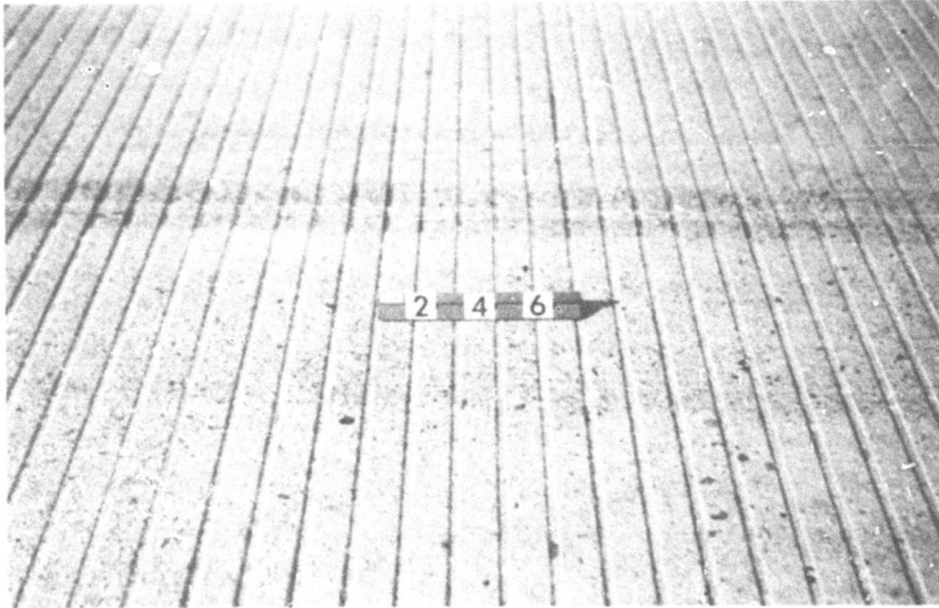
Figure 19. J. F. Kennedy International Airport -- Excellent condition of grooving in northeast end of runway.
