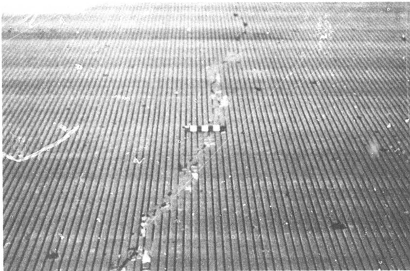
Figure 4. Kansas City Municipal Airport -- Transverse crack and surface voids located in PCC, 1500 feet from north end of runway.
