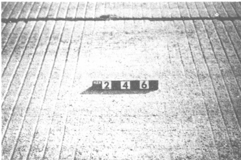
Figure 15. J. F. Kennedy International Airport -- Ungrooved area due to low place in pavement surface.
