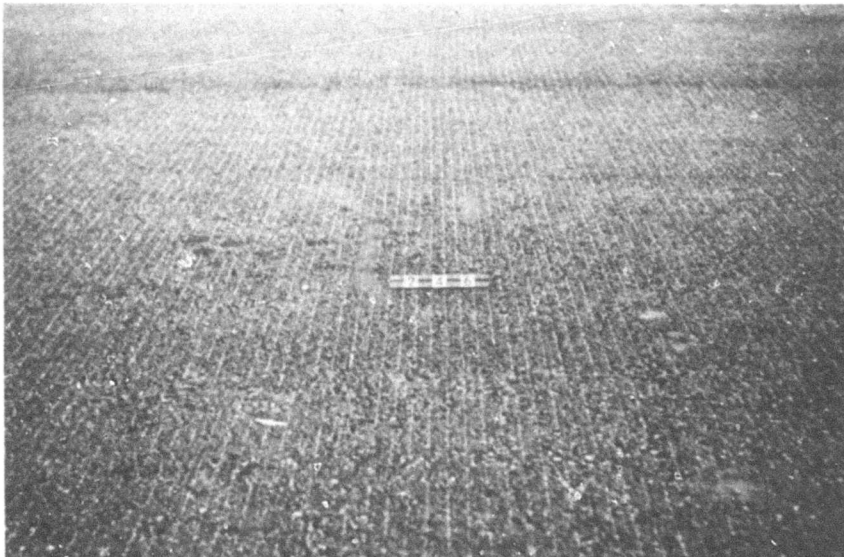
Figure 30. Washington National Airport -- Typical view of AC grooving near south end of runway.
