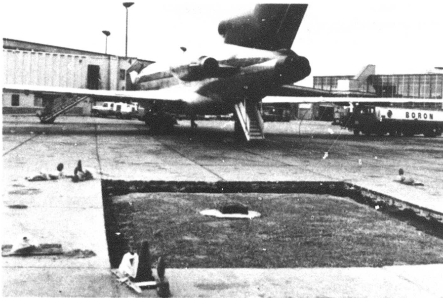
Figure 5. Wirand Concrete Placement Around Drain Box on Apron Slab at Gate Area
