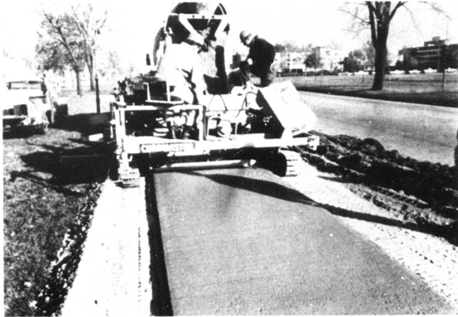
Figure 9. Sidewalk Slipform Paver
