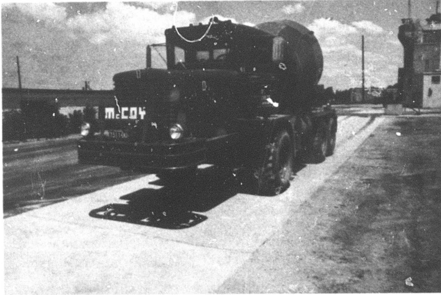
Figure 3. Wirand Concrete Roadway Coming Out of a Ready Mix Plant in Niles, Michigan. Roadway Made Up of Eleven Different Test Sections
