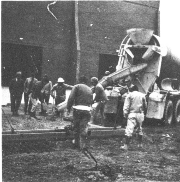
Figure 3. Highlight of the conference visit to CERL was the opportunity to view an actual placement of a 3-in. thick, 35 x 50-ft parking slab constructed on grade with ready-mix fibrous concrete.
