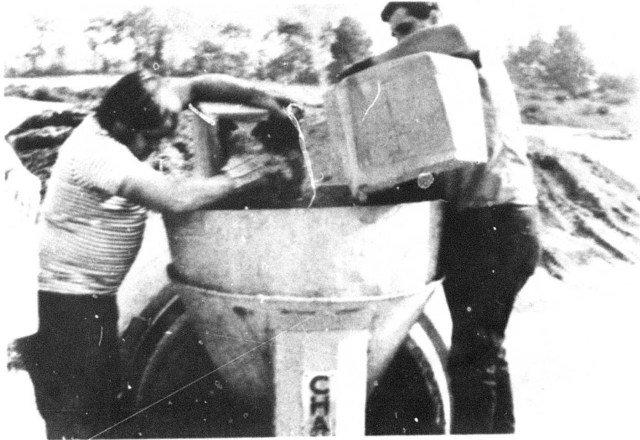
Figure 3. Method 2 Used to Introduce Steel Fibers in the Concrete Batching Operation
