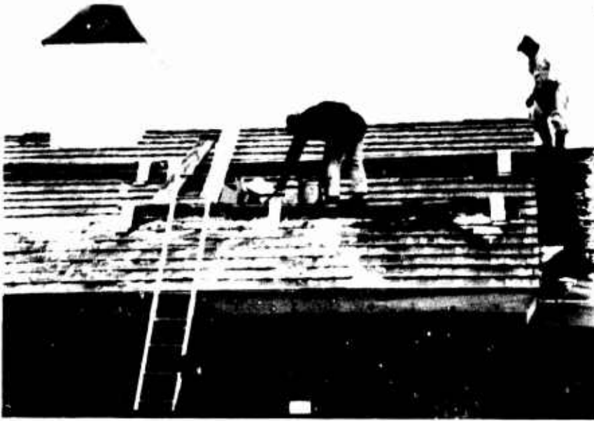
Figure 12. Trial Installation--Light Commercial Construction
