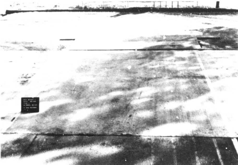
Figure 4. Condition of 6-in. Fibrous Concrete Test Item After 200 Traffic Loadings
