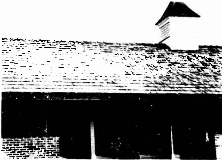
Figure 13. Trial Installation--Light Commercial Construction
