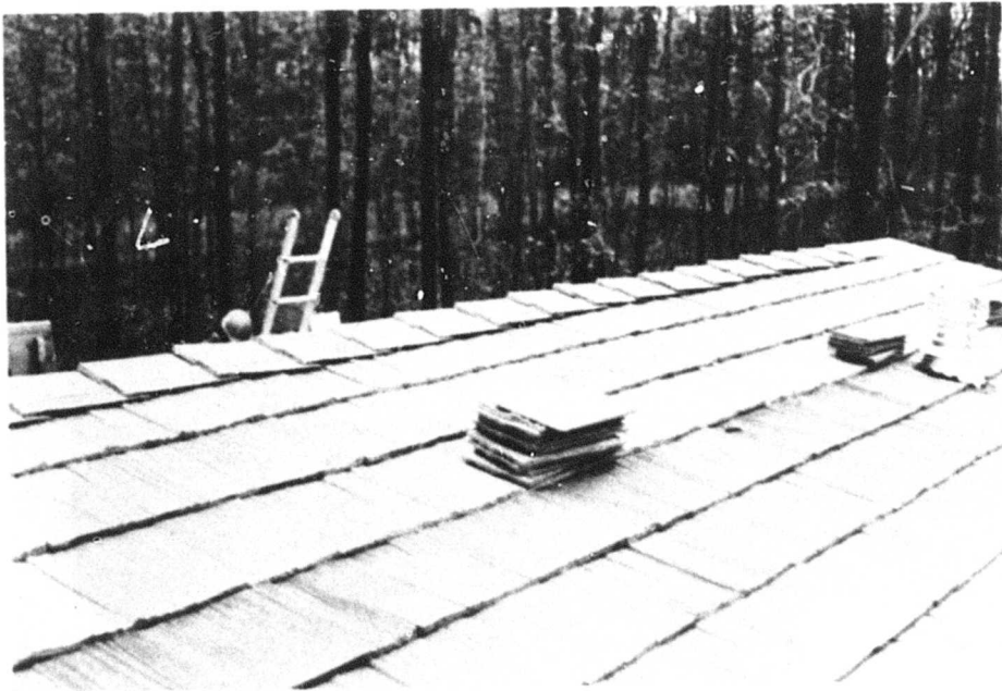
Figure 11. Trial Installation--Residential Construction
