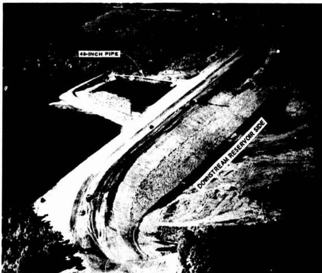
Fig. 3. Island Creek Dam from the downstream (reservoir) side. The 48-in. pipe, shown in the upper center, was used to discharge water through the cofferdam and conduit after closure of the dam during final stages of construction
