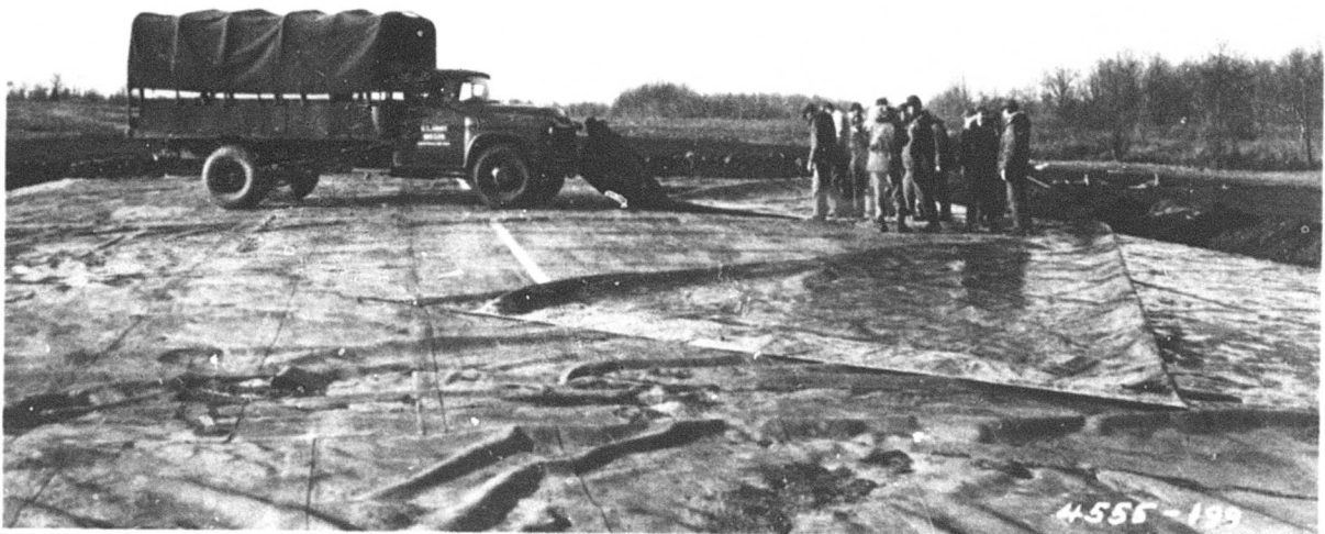
Figure VI-4. Truck pulling membrane section loose from adhesive construction joint.
