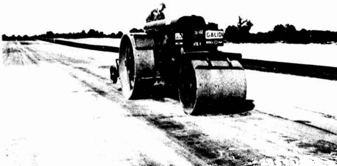
Figure VII-1. Rolling out ruts in soil subgrade beneath membrane surfacing with steel-wheel roller.
