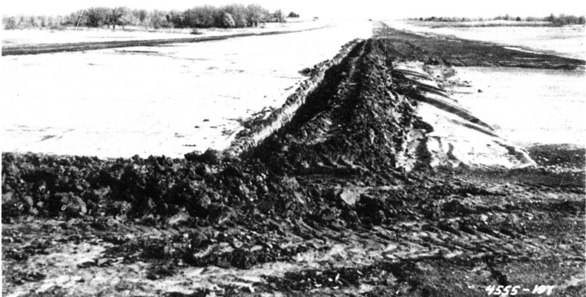
Figure VI-2. Backfill left adjacent to membrane surfacing after the motor grader had removed the soil from the side anchor ditch.
