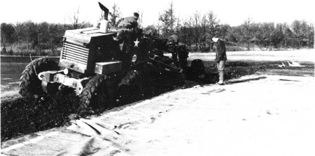
Figure VI-1. Motor grader removing soil backfill from end anchor ditch.
