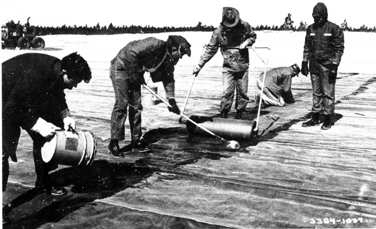
Figure IV-11. Reinforcing adhesive construction joint with a 36-in.-wide strip of membrane.
