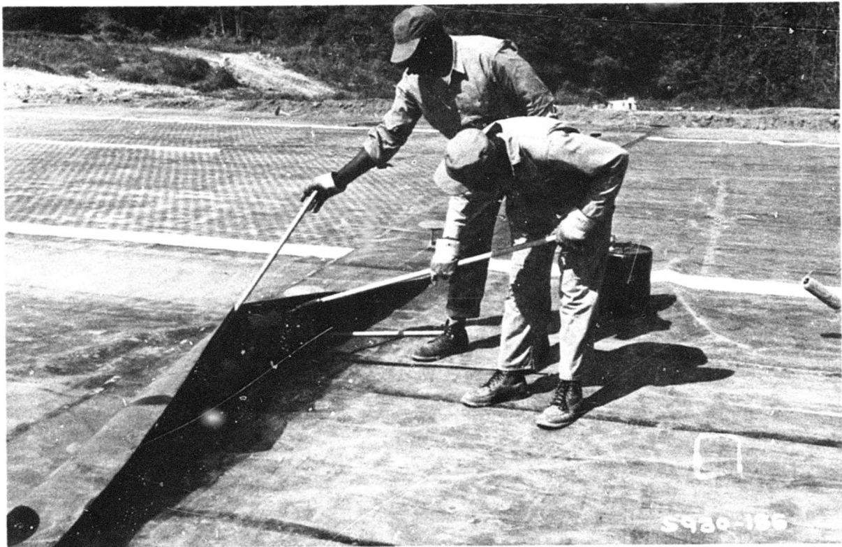
Figure IV-10. Overlapped end of second section raised with 48-in.-long paint roller handles.
