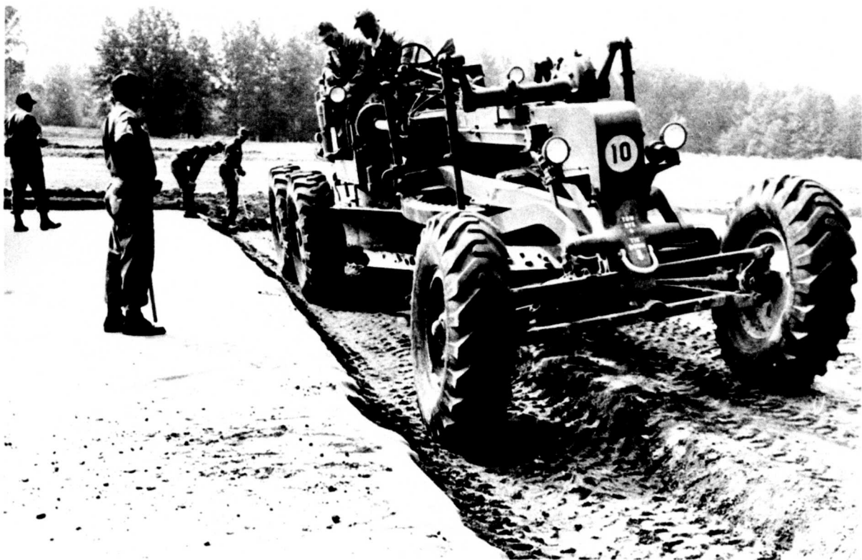
Figure IV-15. Compacting backfilled anchor ditch with motor grader.
