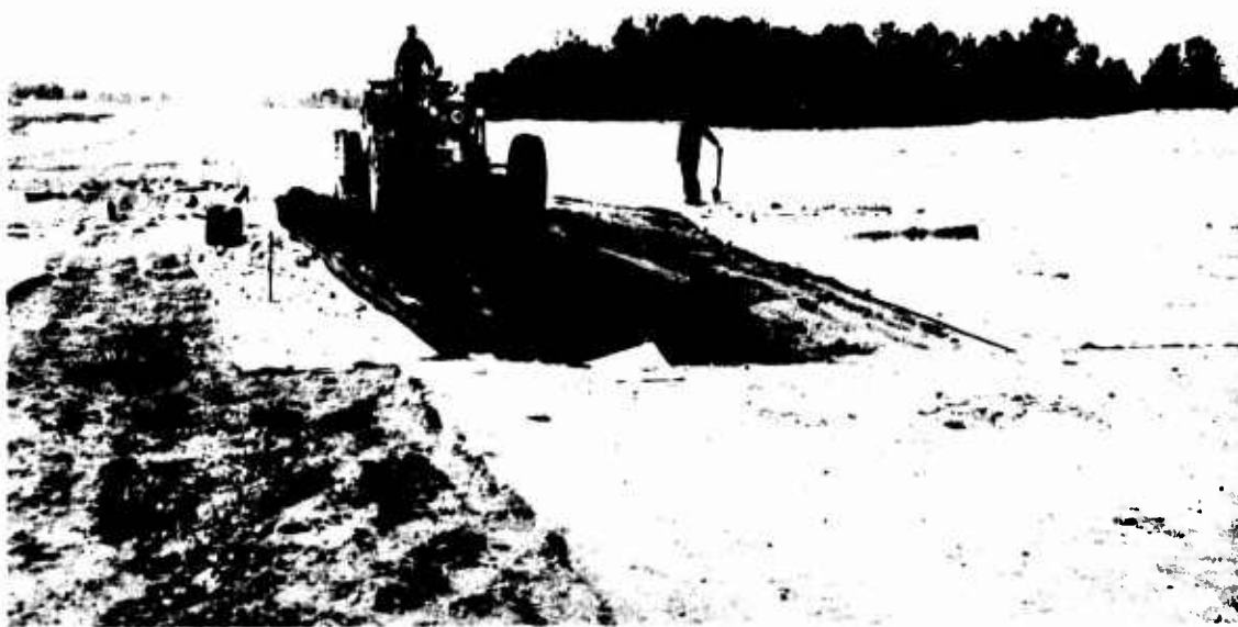
Figure VII-2. Motor grader spreading backfill material in rutted area.
