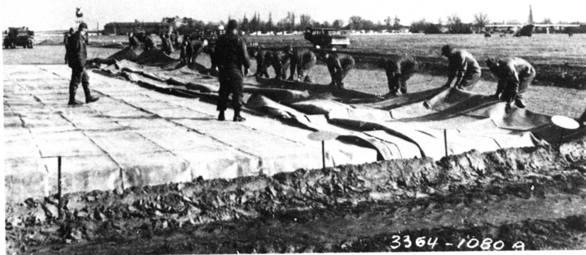
Figure IV-3. Troops stationed along edge of surfacing unfolding it into side anchor ditch.
