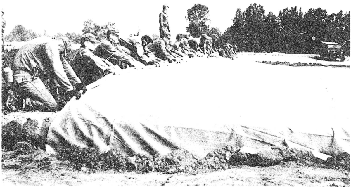
Figure IV-5. Troops removing slack from section of surfacing by pulling on free end of surfacing.
