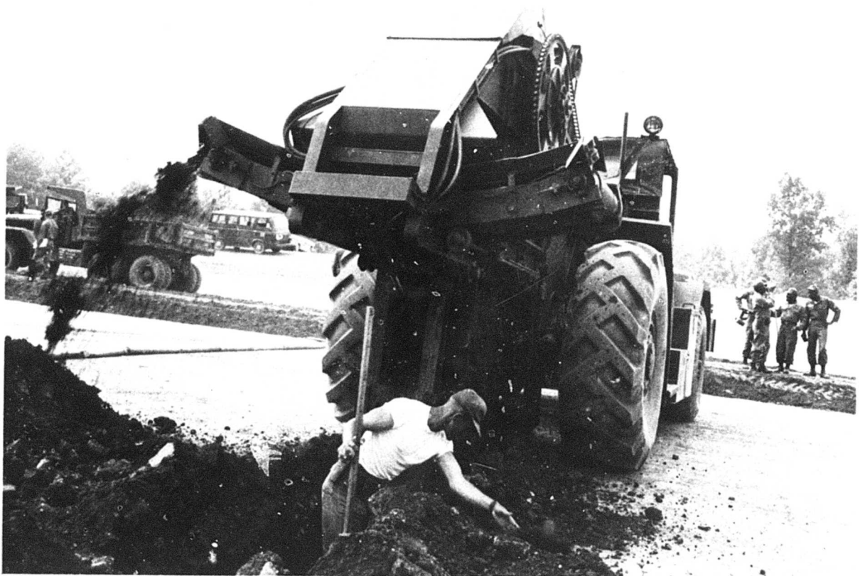
Figure III-2. Ditching machine constructing 2-ft-deep anchor ditch.
