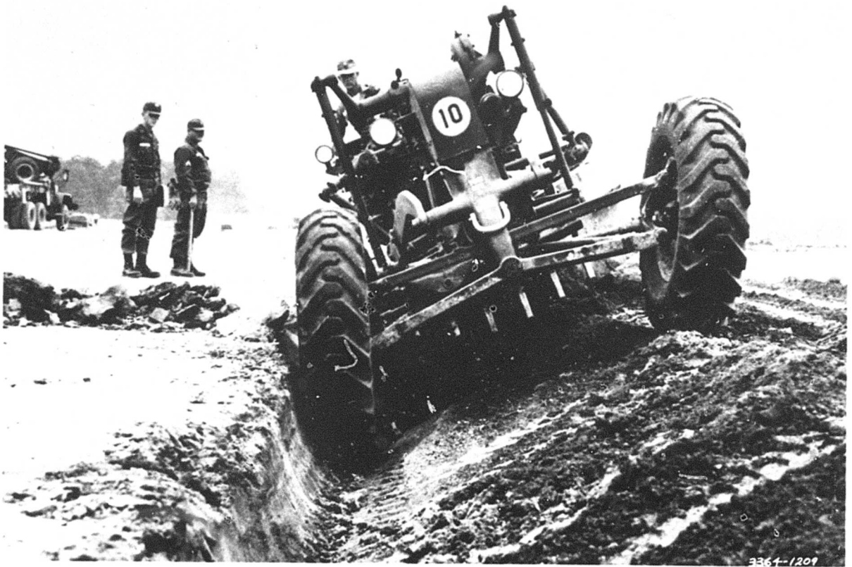
Figure III-1. Motor grader constructing L-shaped, 2-ft-deep anchor ditch.
