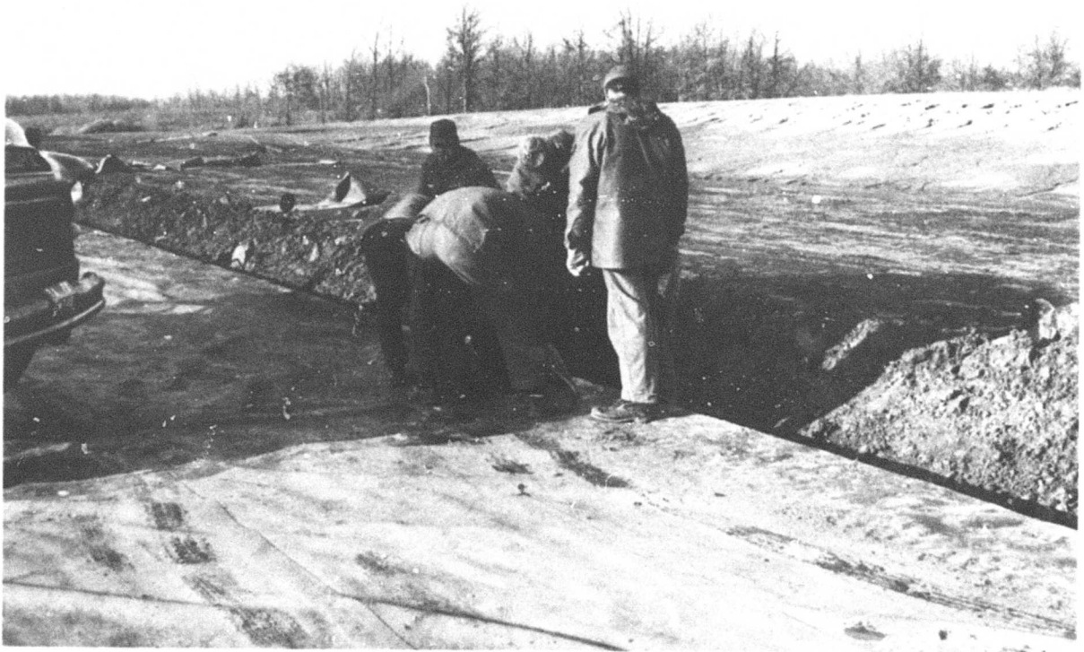
Figure VI-3. Troops peeling corner of adhesive construction joint loose.
