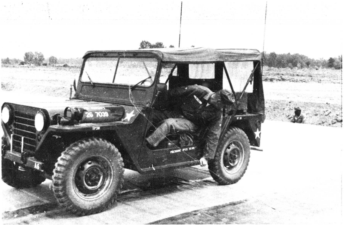
Figure IV-12. Rolling adhesive construction joint with jeep.
