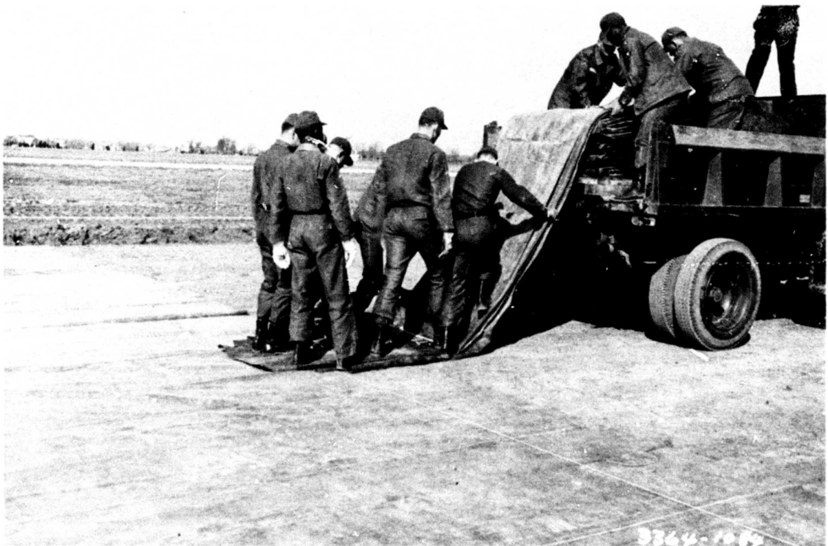
Figure IV-8. Second section of surfacing overlapping first section approximately 24 in.
