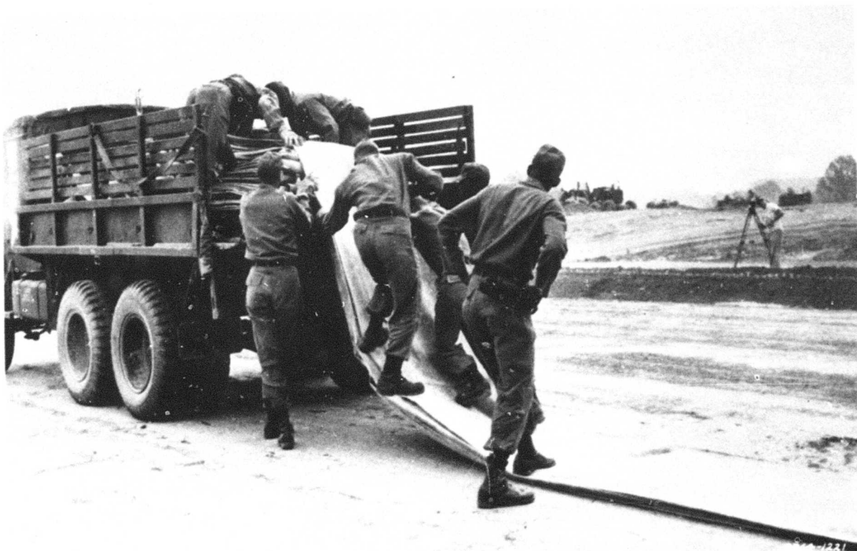
Figure IV-2. Unfolding membrane from truck onto ground along center line of area to be surfaced.
