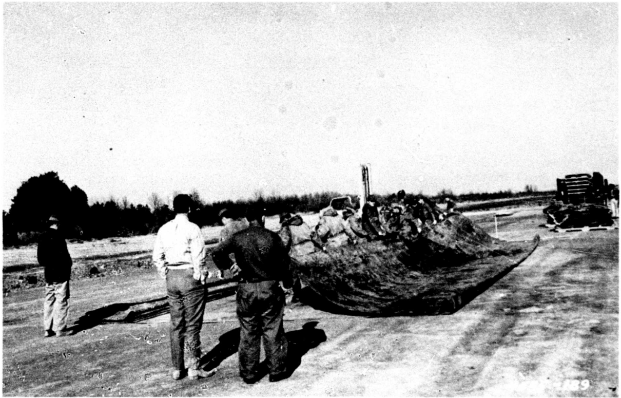
Figure VI-5. Troops accordion-folding membrane section.
