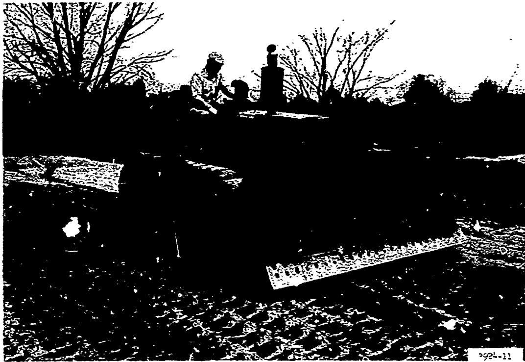
Photograph 4. Spreading sand in item 2 with D4 tractor
