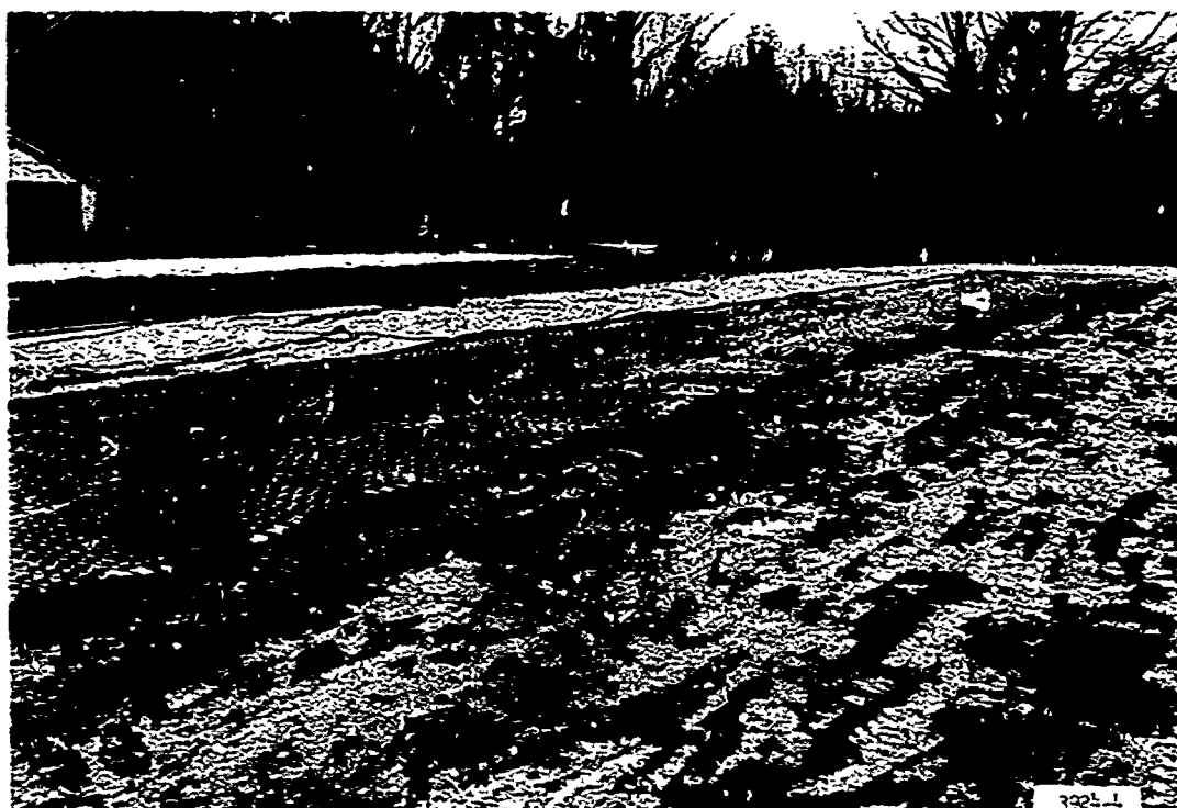
Photograph 2. Deteriorated M6 landing mat surface
