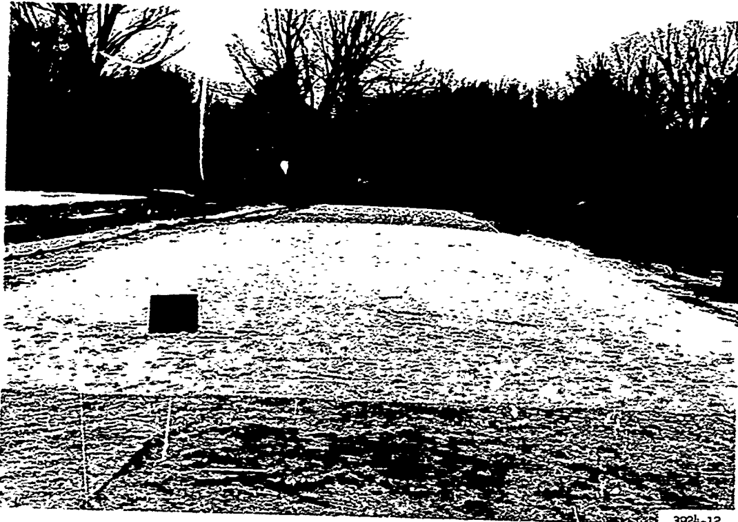
Photograph 5. Test section after construction of overlay soils
