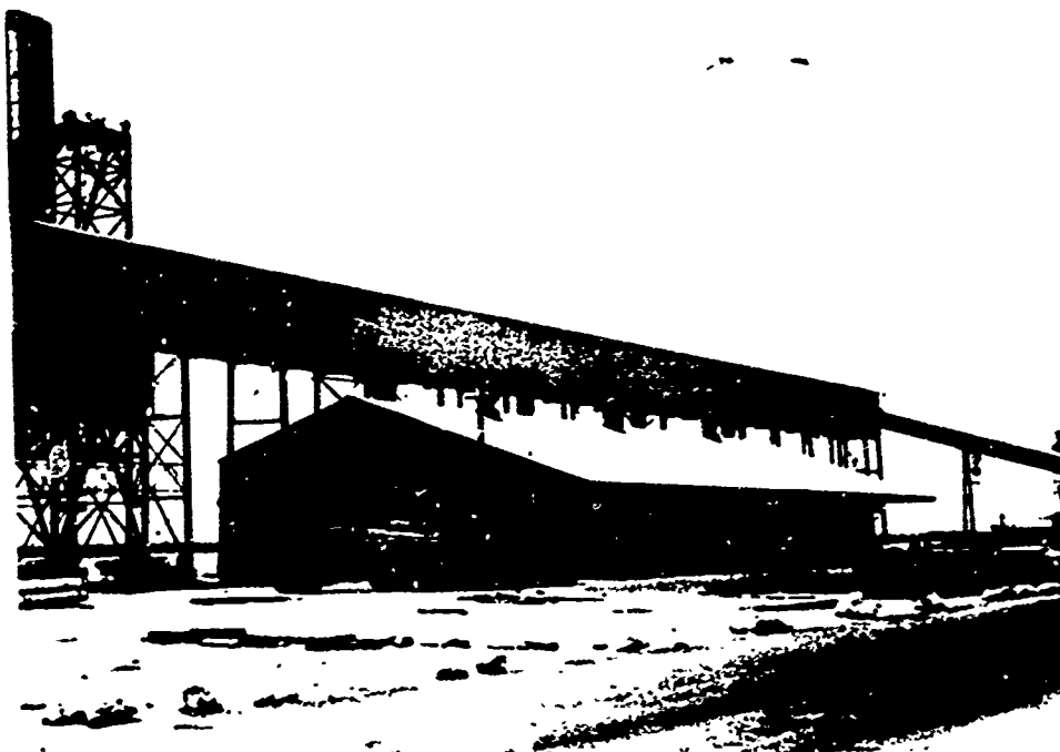
Fig. 115. Sugar conveyor and terminal facility, Phases I and II.
