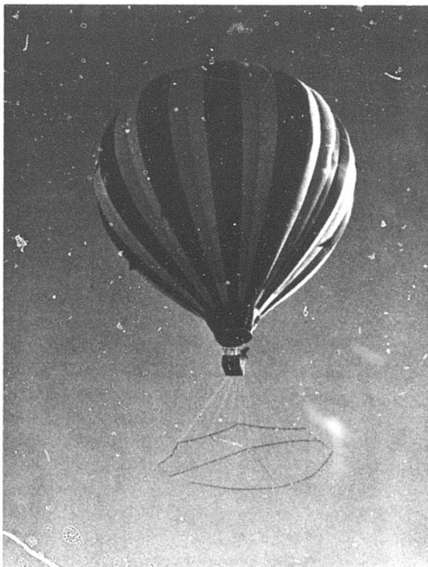
FIG. 12. Spray Assembly Suspended From Balloon.
