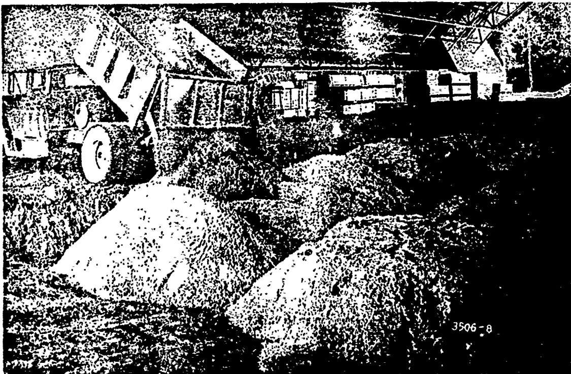
Fig. 4. End-dumping of sand in item 4
