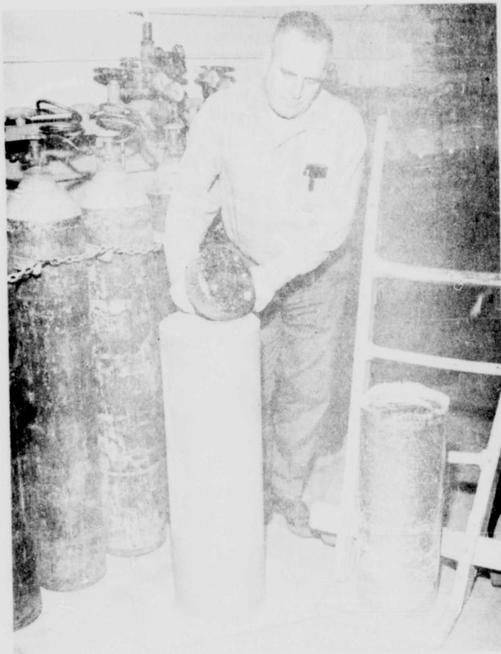
FIGURE 7. - As-cast remelt ingot, crucible, and electrode stub
