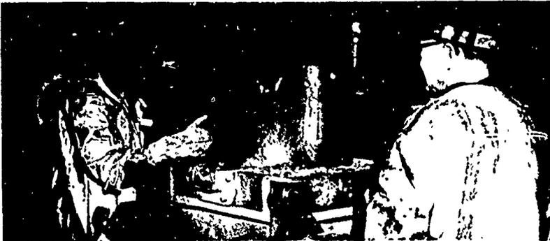
Figure 2. Air-Induction Melting of TRIP Steel Alloy Using Argon Shield. Temperature Reading Being Taken.
