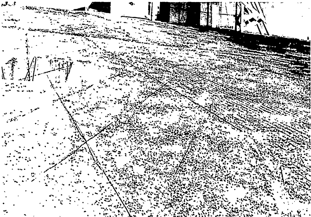
Photo 12. Chopped glass and DCA-1295 in area adjacent to wire mesh
