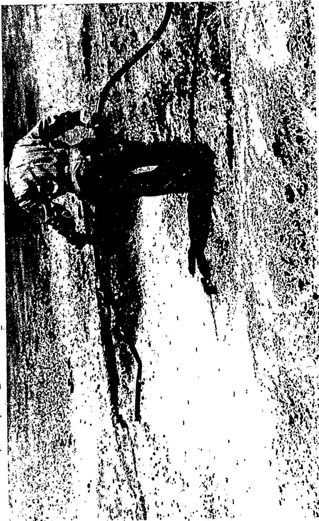
Photo 9. Application of DCA-1295 on an area covered with chopped glass
