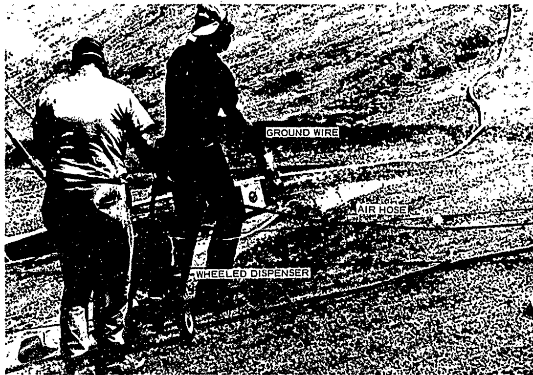
Photo 8. Typical operation showing cutter gun, dispenser, and crew
