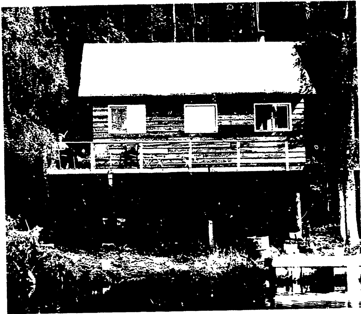
Figure 7.--Two-bedroom house on wood-post foundation from plan 1-489, designed for a vacation house. Built by owner with a material cost of $1,700, including foundation, plumbing, or electrical systems.
