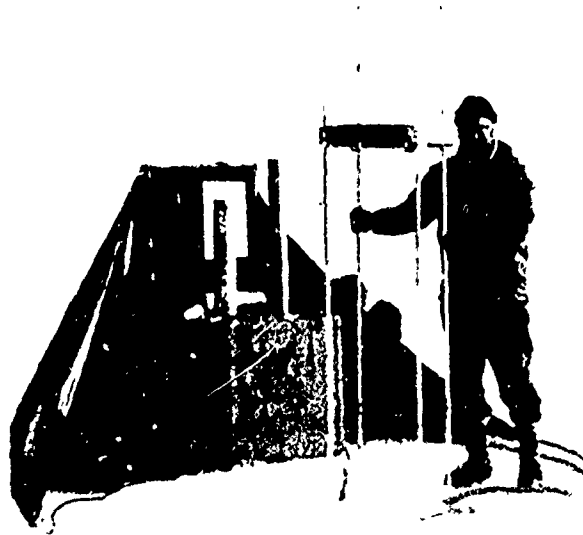
Figure 3a. Inventor R.E. Francois and 100,000 Btu Per Hour Thermal Ice Corer
