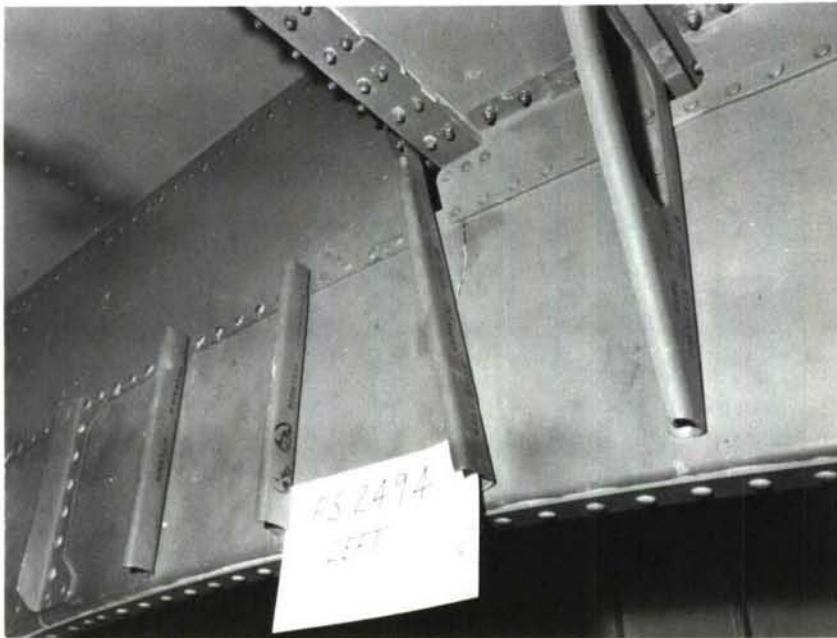
FIGURE 67. FATIGUE DAMAGE AT FUSELAGE FRAME STATION F.S. 2494. LOOKING AFT.
