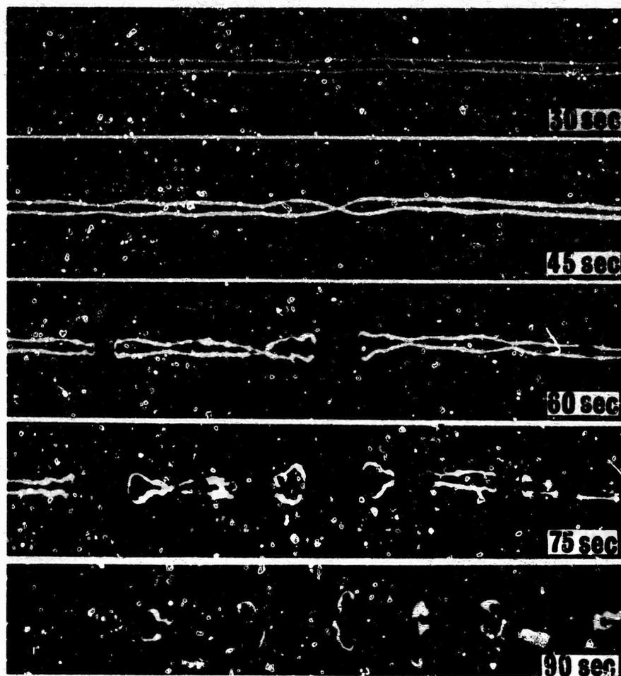
Fig. 1. B-47 CONTRAIL BREAKUP BY SINUOUS INTERACTION OF VORTICES (from Smith and Diamond, 1956, as reproduced by MacCready, 1971)
