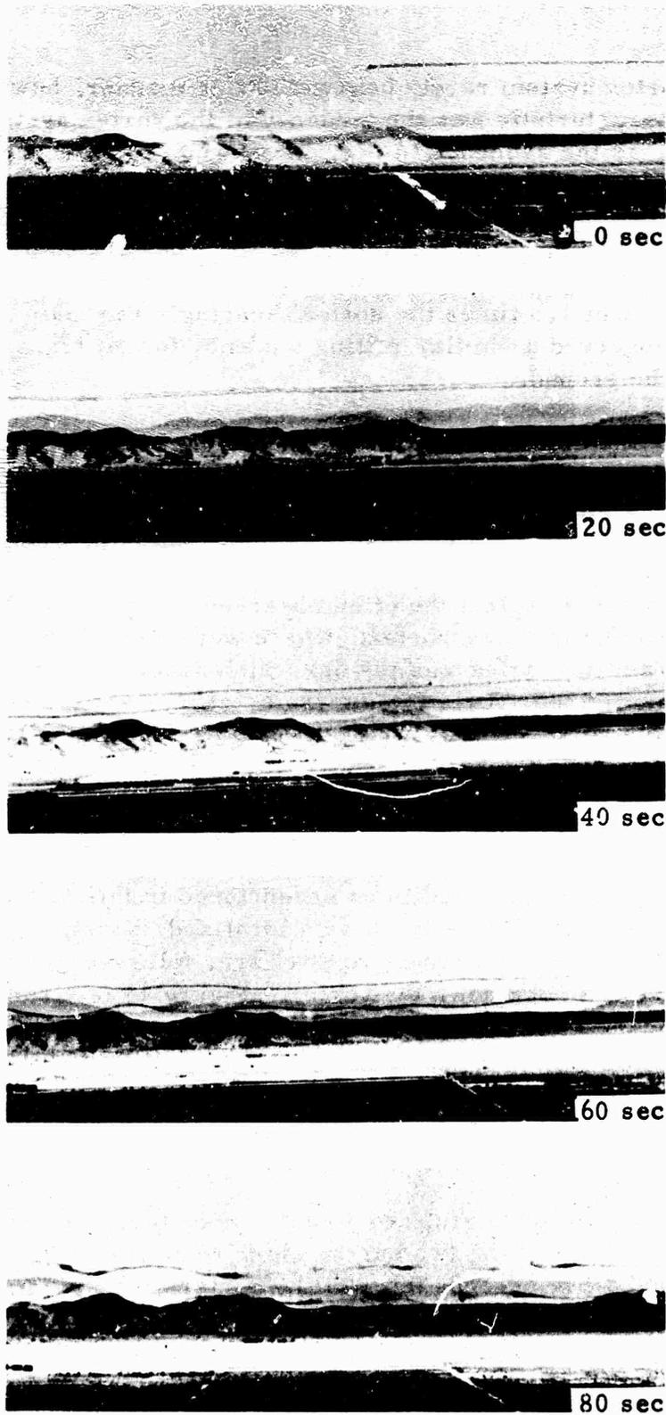
Fig. 14. SIDE VIEW OF WAKE IN CALM, STABLE ATMOSPHERE AT 20-SECOND INTERVALS, SHOWING ROLLING TENDENCY AND DESTRUCTION BY CORE-BURST INSTABILITY
