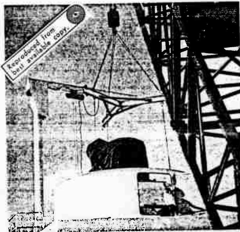
Figure 2-4. Installation of NIKE-AJAX Pedestal
