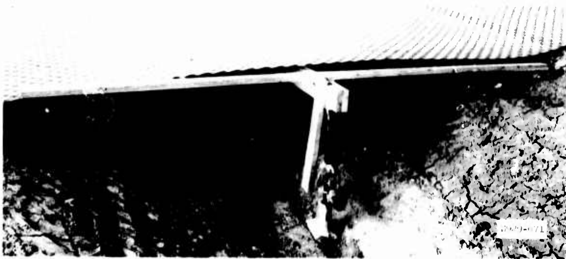
Fig. 12. Frame lifted to eliminate sag in MO-MAT across catenary ditch
