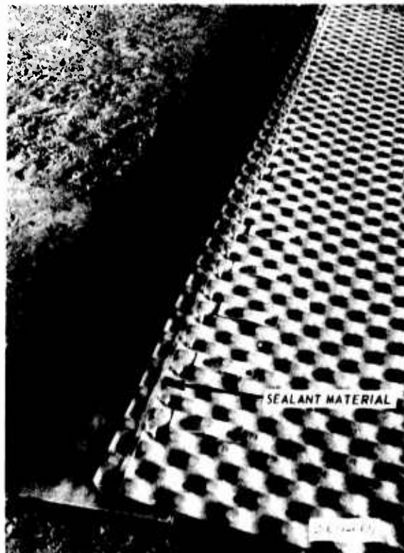
Fig. 7. Underlap panel prior to bolting
