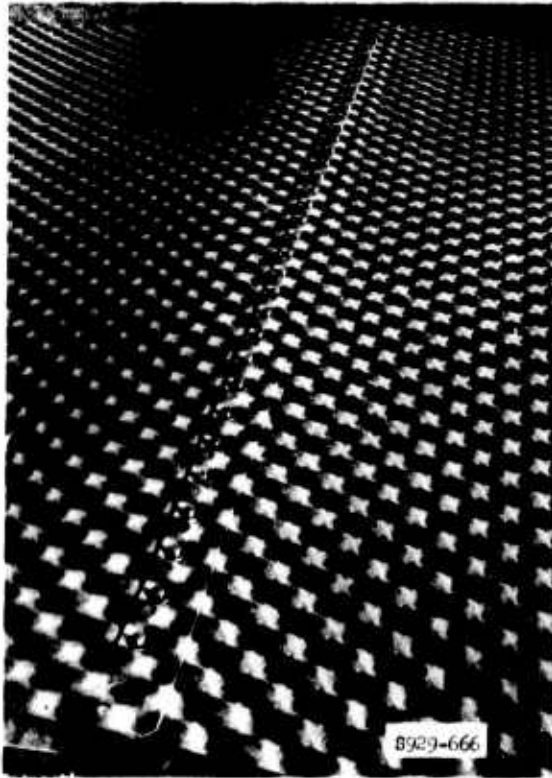
Fig. 8. Typical transverse joint after bolting
