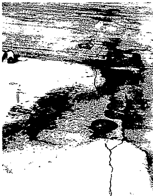
Photograph 57. Burlington Municipal Airport. Typical cracking in epoxy-asphalt pavement
