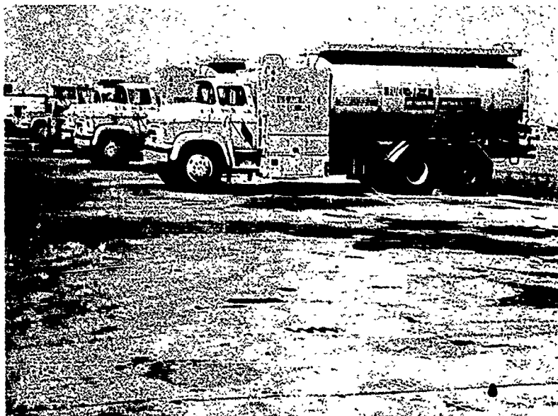
Photograph 9. Bunker Hill AFB. Overlay on flexible pavement used for parking fuel trucks. Note heavy spillage of fuel and oil
