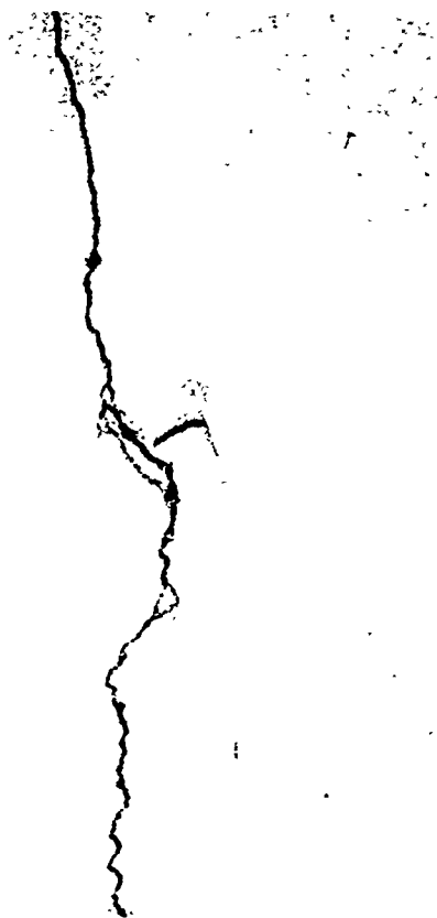
Photograph 40. Reno ANG Field. Close-up showing fragment of pavement broken out of epoxy- asphalt overlay
