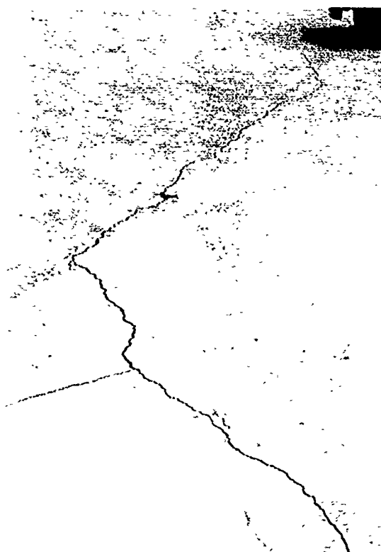
Photograph 40. Reno ANG Field. Close-up showing fragment of pavement broken out of epoxy- asphalt overlay
