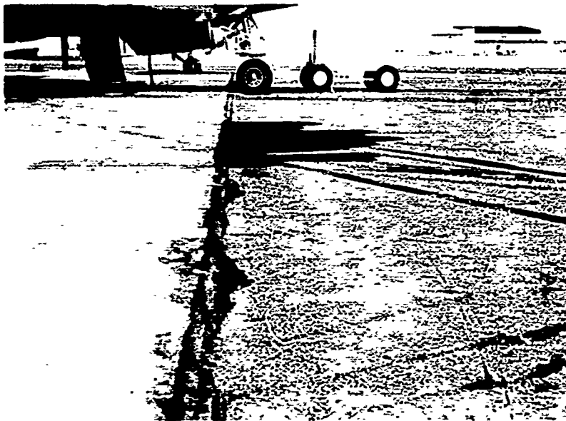
Photograph 1. Berry Field. Edge of overlay pavement. Note proximity of joint in original pavement
