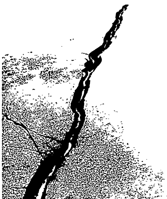
Photograph 43. Seymour Johnson AFB. Crack sealed with emulsion
