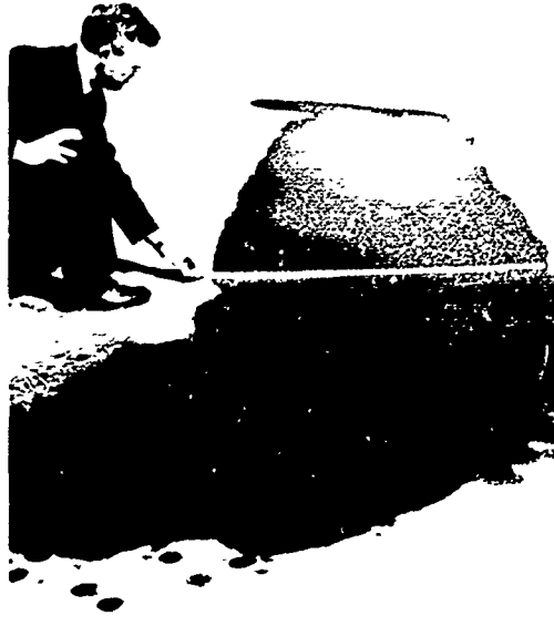
Photograph 50. Hancock Field. Fuel spillage on epoxy-asphalt pavement.
