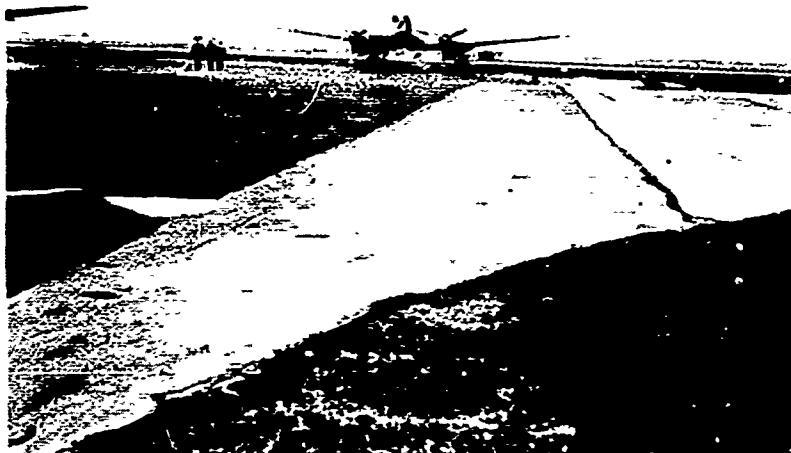
Photograph 5. Wright-Patterson AFB. Overlay at transition from taxiway to apron
