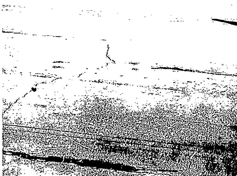
Photograph 53. Bradley Field. Transverse crack patterns. The white line is parallel to the center line of the runway
