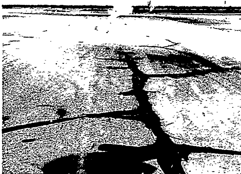
Photograph 23. Davis-Monthan AFB. Unsuccessful attempts to seal cracks in epoxy-asphalt pavement
