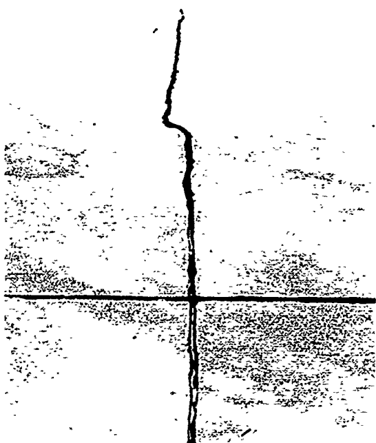
Photograph 42. Seymour Johnson AFB. Cracks that have been routed and sealed with epoxy asphalt
