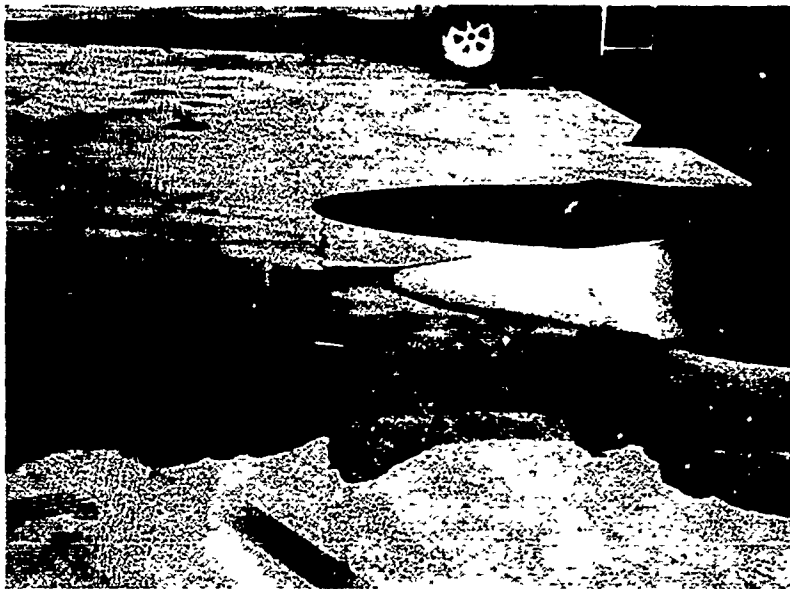
Photograph 15. Truax Field. Profuse fuel spillage. Note flow over reflection crack
