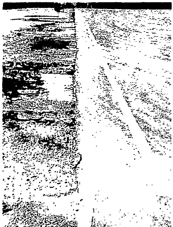
Photograph 18. Perrin AFB. Cracking parallel to paving lane
