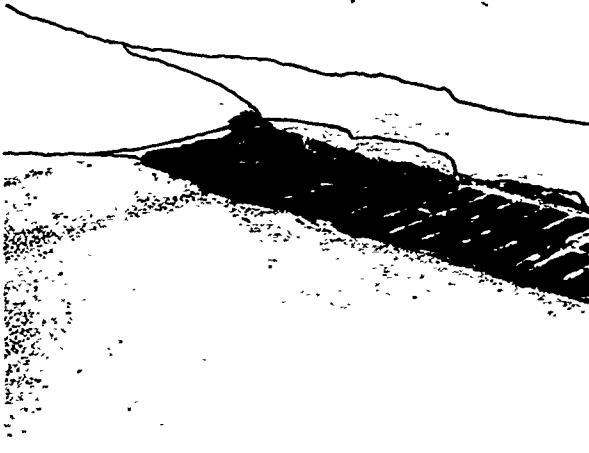
Photograph 49. Hancock Field. Cracks around drop-inlet drain. Cracks retouched on photograph to make them more visible
