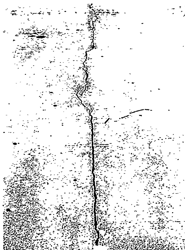
Photograph 54. Bradley Field. Open construction joints in the epoxy-asphalt pavement
