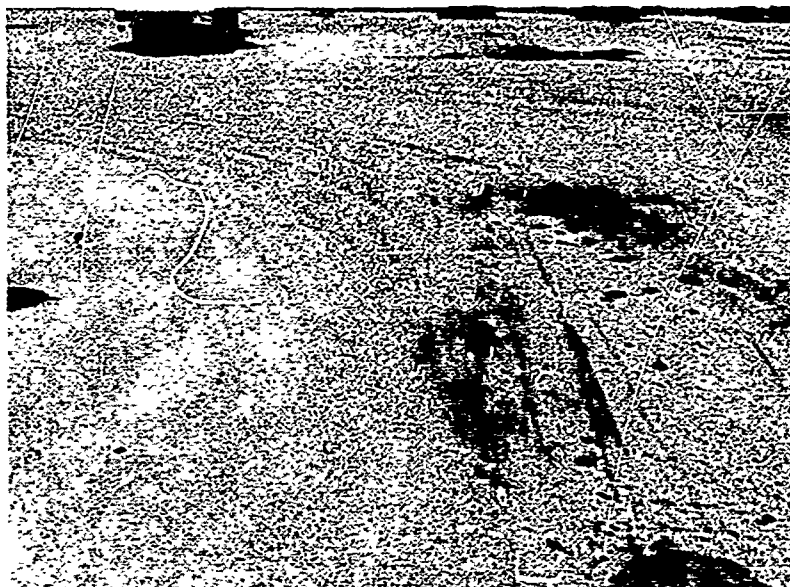
Photograph 21. Perrin AFB. Surface disintegration due to saturated underlying pavement
