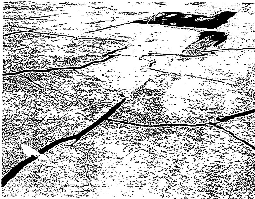
Photograph 64. Westchester County Airport. Cracking pattern on epoxy-asphalt pavements with patches in background
