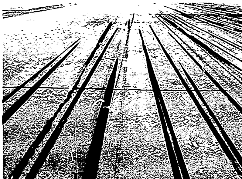
Photograph 27. George AFB. Reflection cracks which had been sealed
