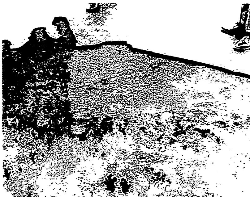
Photograph 62. Loring AFB. Area where outboard engine of a B-52 had blown away a small portion of epoxy-asphalt pavement
