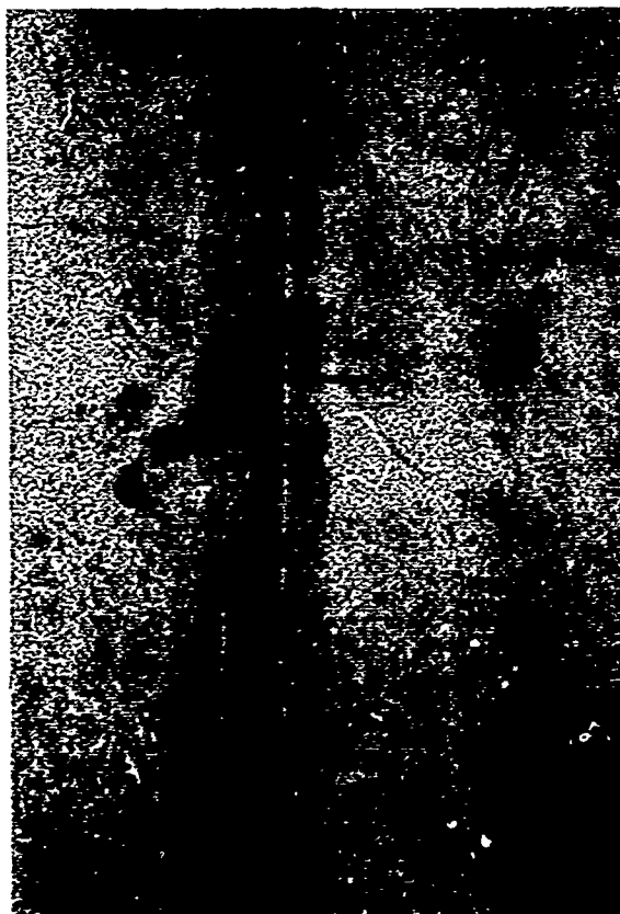
Photograph 32. George AFB. Blisters in pavement containing water
