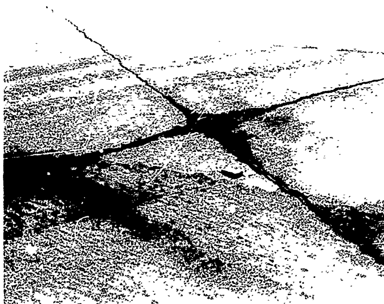
Photograph 44. Seymour Johnson AFB. Cracks in epoxy- asphalt pavement. Note joint-filling material in cracks in foreground
