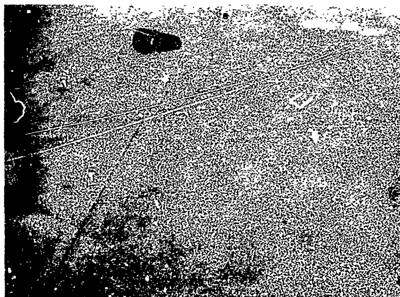
Photograph 38. Reno ANG Field. Close-up of epoxy-asphalt overlay surface
