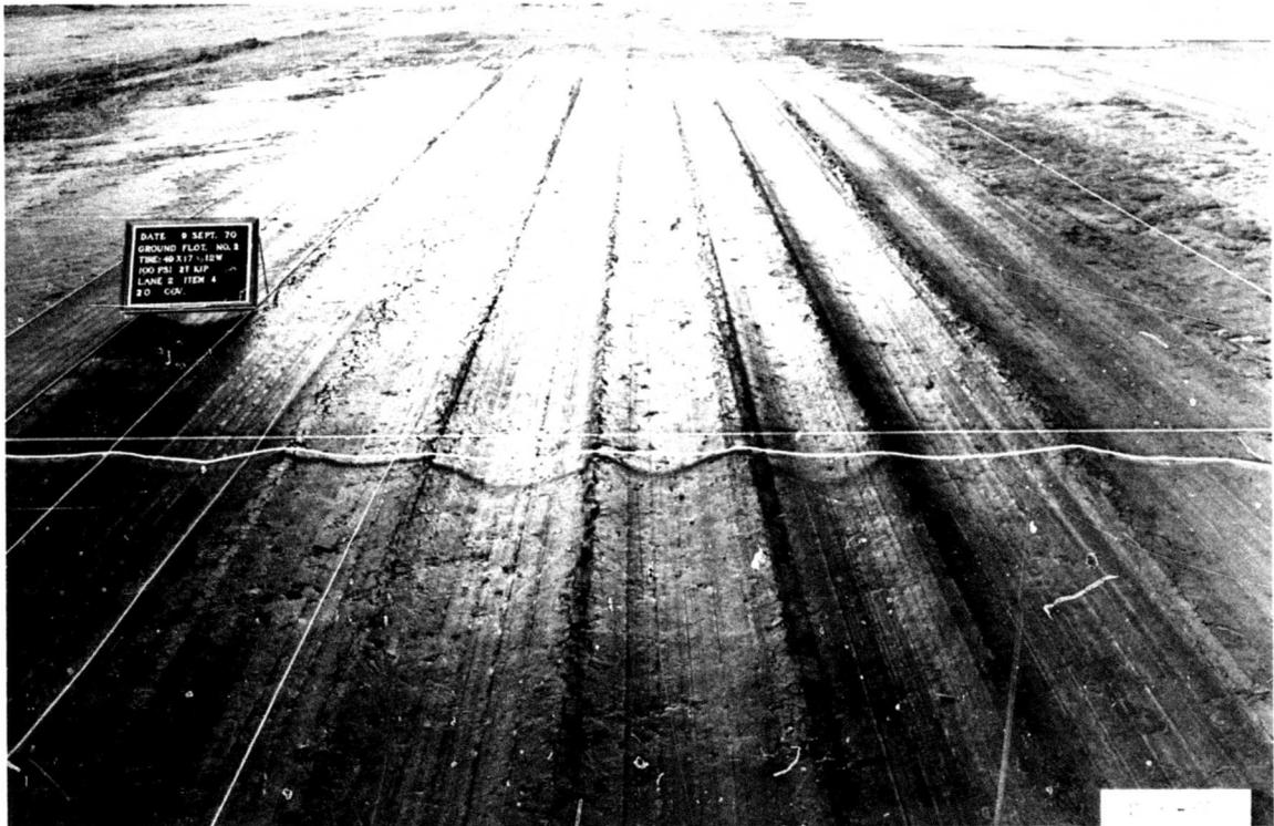
Photo 18. Test section 2, lane 2, item 4, at failure after 20 coverages
