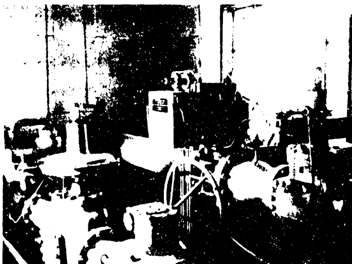
Interior of Regulator Building showing Regulators and Hi-Low Operators. Looking towards ground zero.
