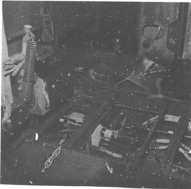
Figure 20. Full View of Vortex Valve Servoactuators Installation.
