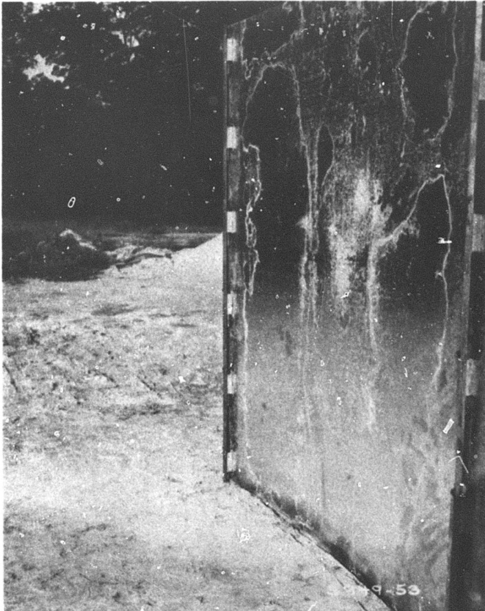
Photograph 21. Sheets of ARMCO I connected by pins
