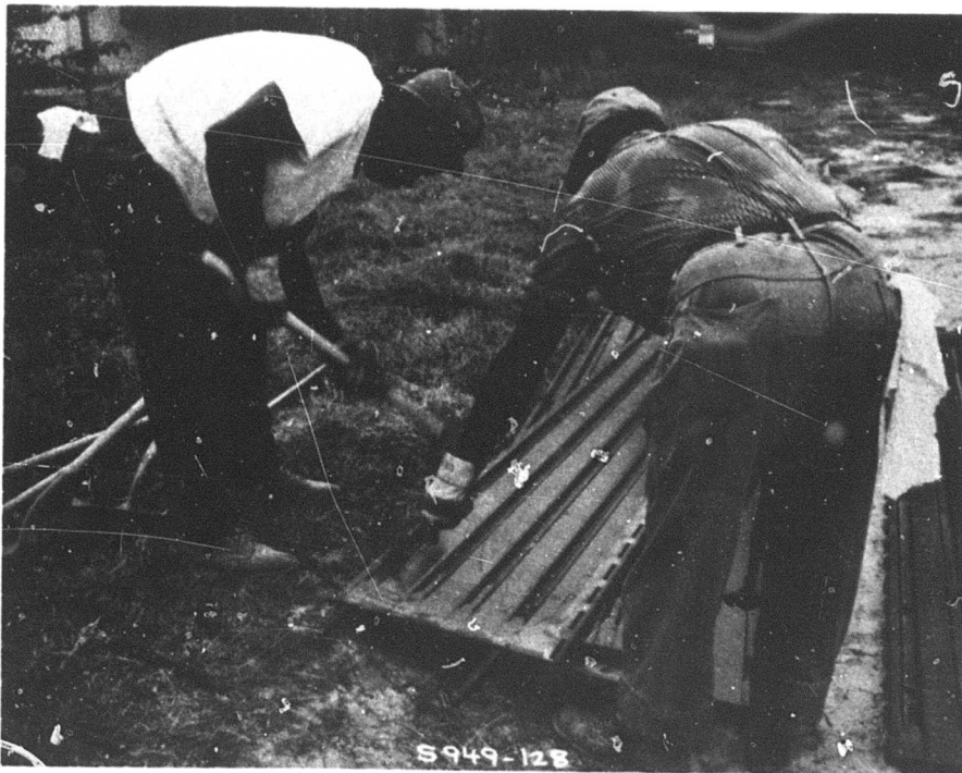
Photograph 67. Removing locking pins to clear frame of M8A1 mat
