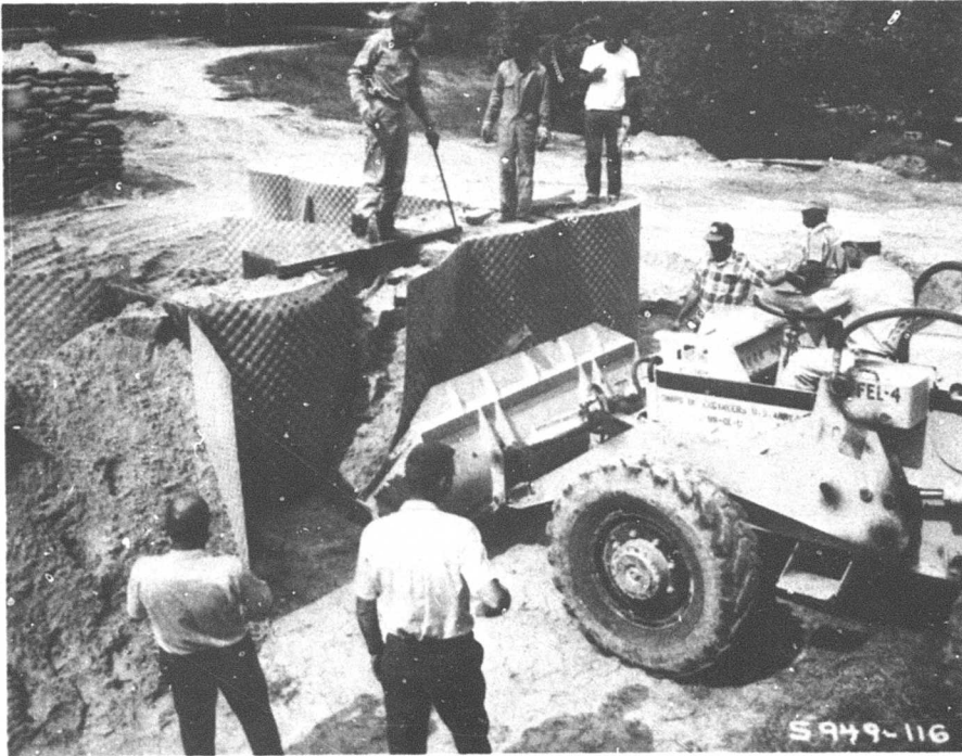
Photograph 13. Disassembly of Air Logistics II revetment
