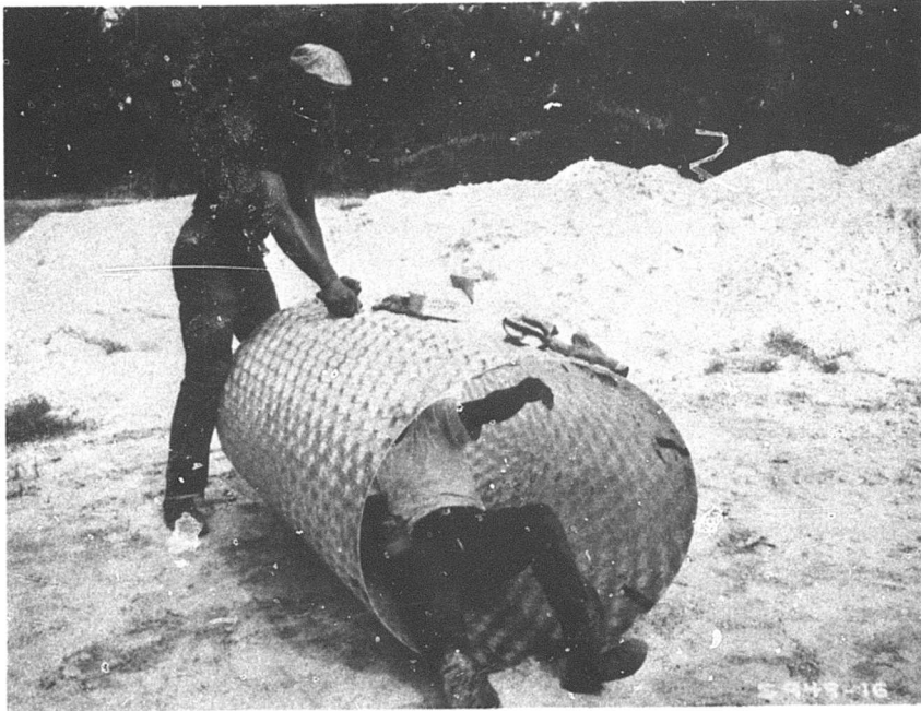
Photograph 3. Bolting MO-SHEL cylinder
