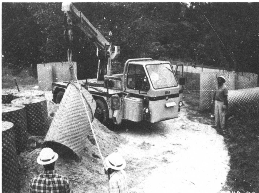
Photograph 8. Truck-mounted crane emptying MO-SHEL cylinders
