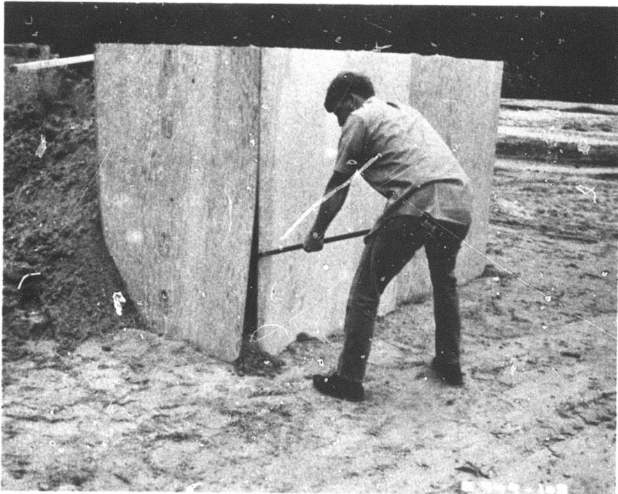
Photograph 65. Disassembly of plywood revetment
