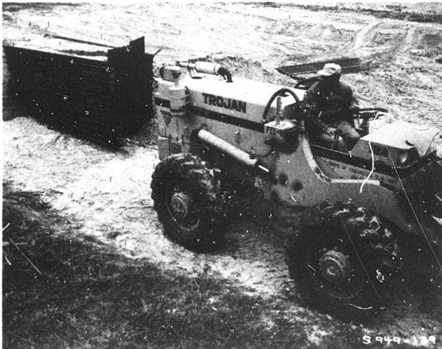
Photograph 77. Disassembly of M8A1 revetment using sheet metal clamp
