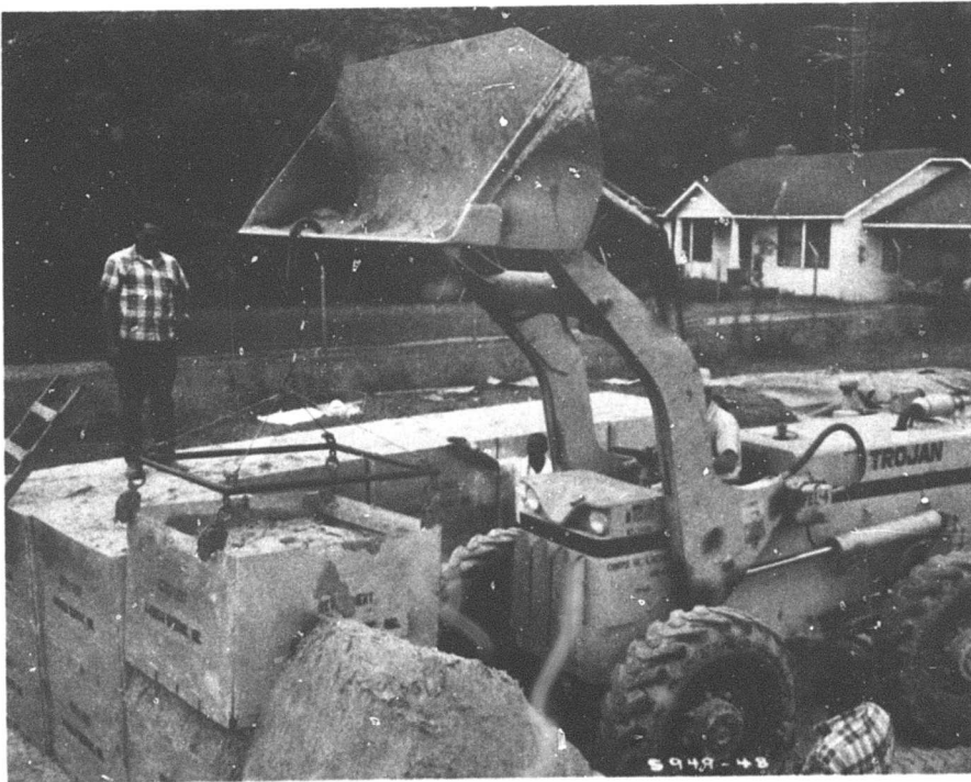
Photograph 19. Spreader bar being used to disassemble AEI revetment
