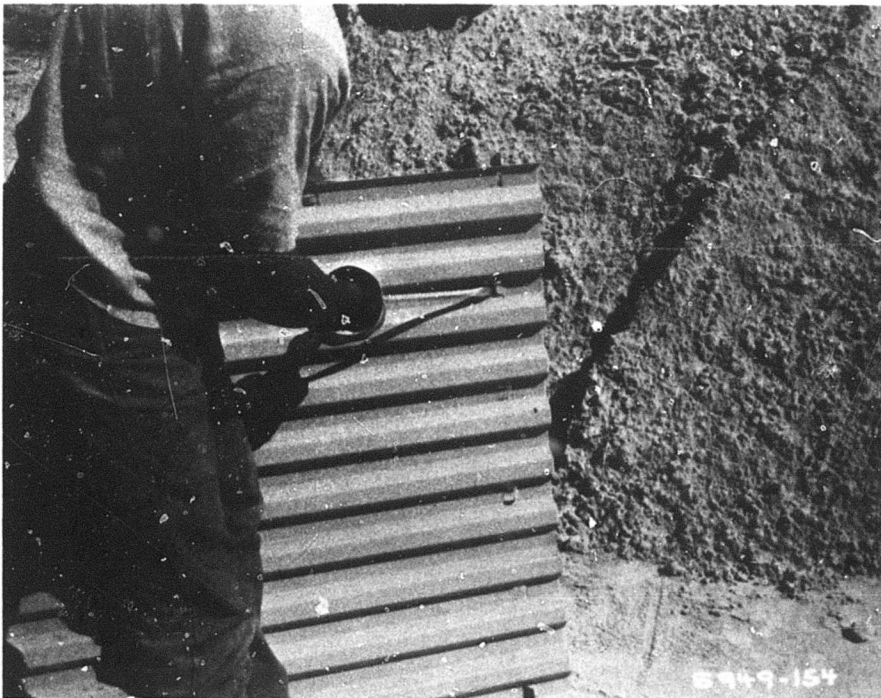
Photograph 79. Banding ground mat tab to accept frame
