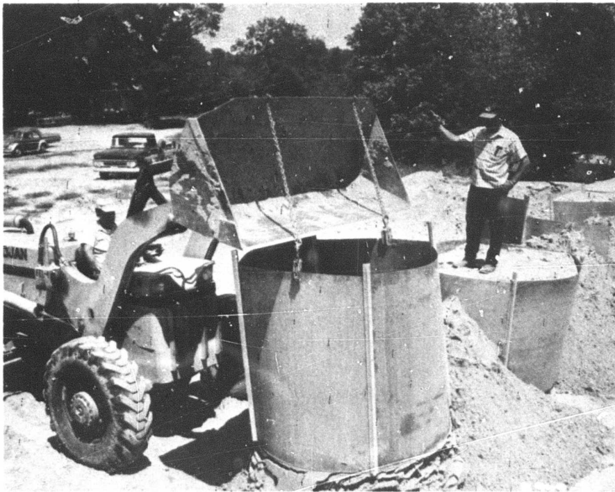
Photograph 33. ARMCO II disassembly operations
