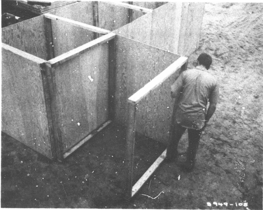
Photograph 64. View of right-angle turn in plywood revetment
