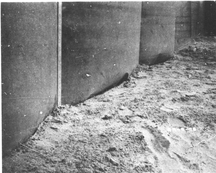
Photograph 31. Buckling of 20-gage ARMCO II paneling at bottom of revetment
