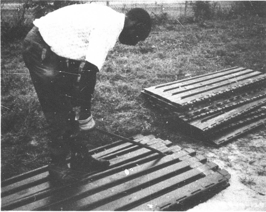
Photograph 68. Bending tabs to clear frame of M8A1
