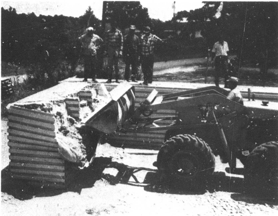
Photograph 59. Disassembly of Republic Steel revetment
