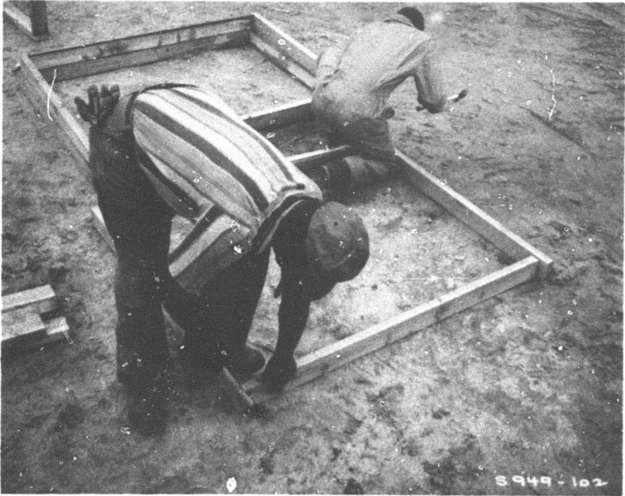
Photograph 62. Assembly of timber framework for plywood revetment
