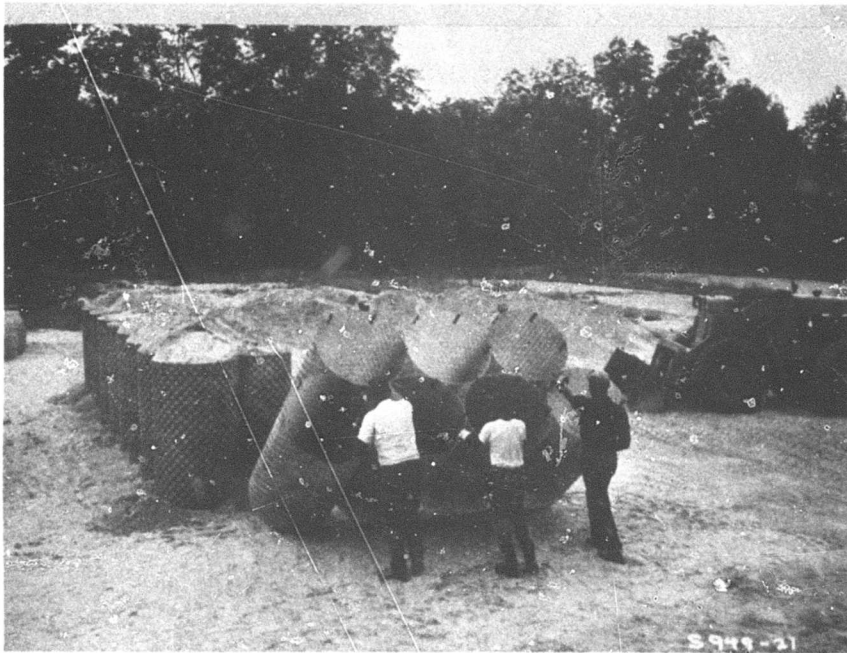
Photograph 5. Forming MO-SHEL cylinder wall
