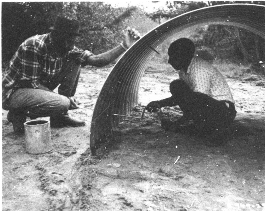
Photograph 37. Joining Kaiser Aluminum culvert halves
