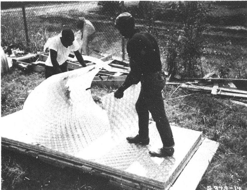
Photograph 2. Rolling MO-SHEL into a cylinder
