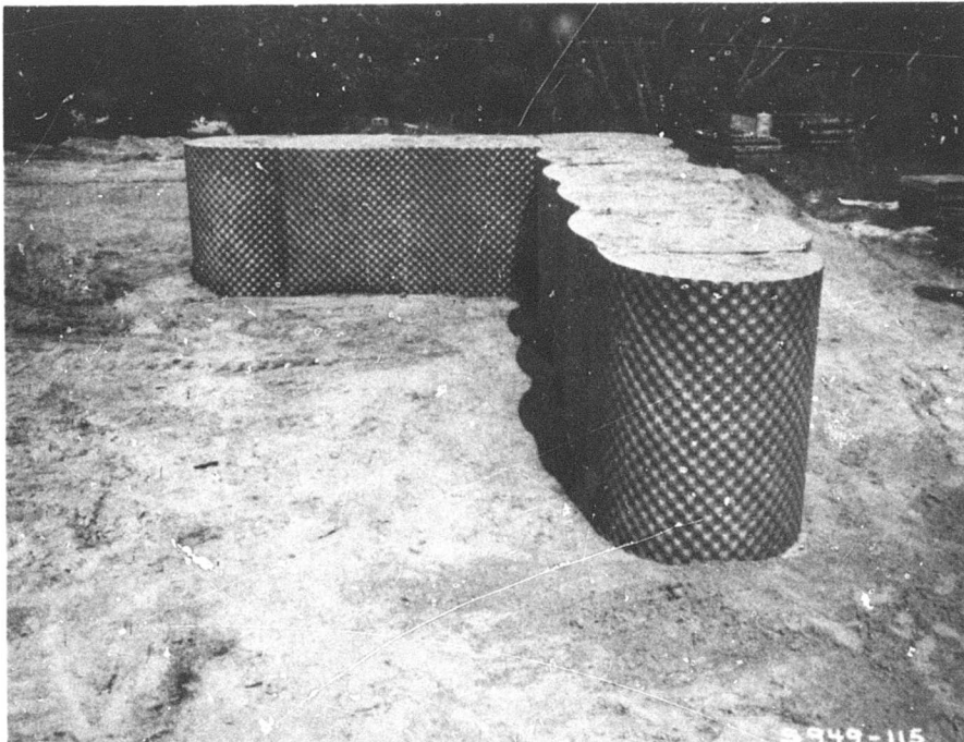
Photograph 12. Completed Air Logistics II revetment
