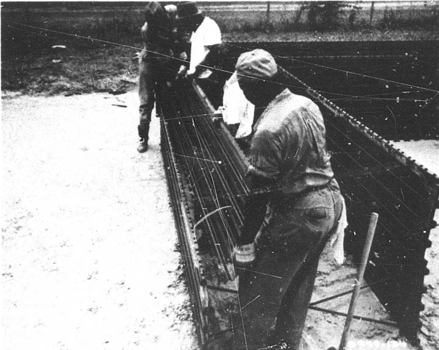
Photograph 73. MSA1 assembly operation, connecting panels
