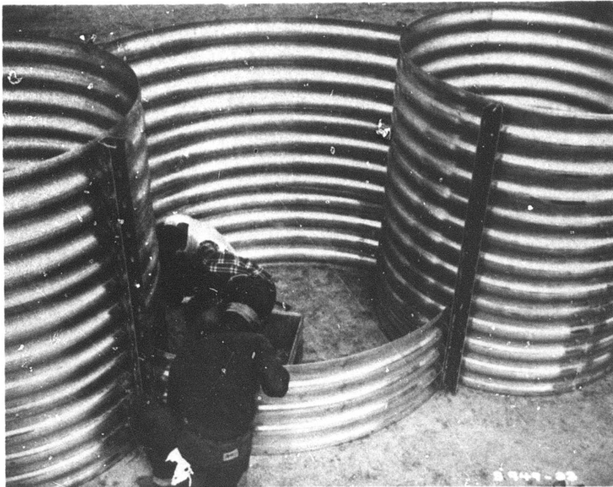
Photograph 39. Assembly of Kaiser Aluminum arch sections
