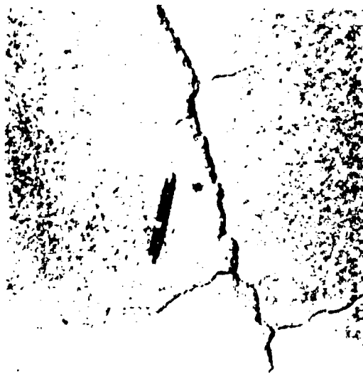
Photograph 3. Typical cracks in untreated pavement
