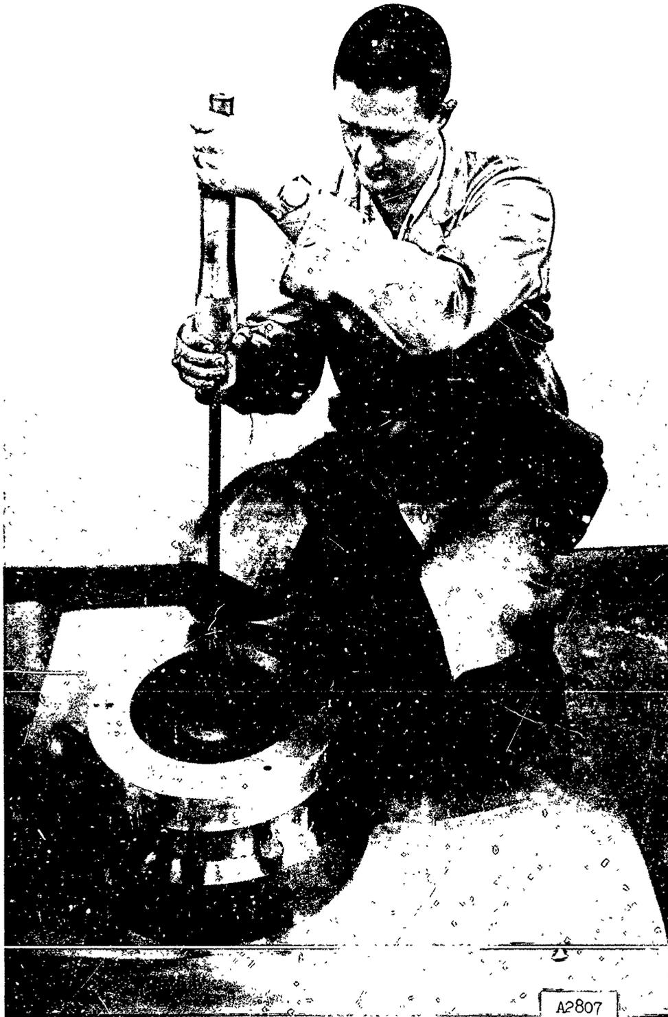
Fig. 7. Dynamic compaction of cohesive specimen
