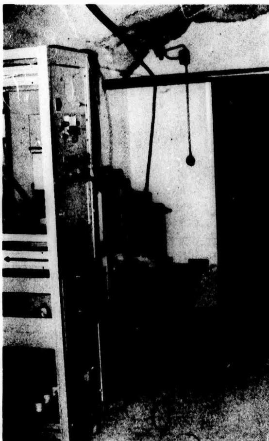
PLATE 4: The high-gain control panel, located in the front section of the tunnel, is in the foreground. The wooden covered cable trough is visible at the middle right of the picture just in front of the door. Power cables run along the ceiling, which is covered with shotcrete. The chart recorder was used during the high-gain installation. The view is aimed approximately south.
