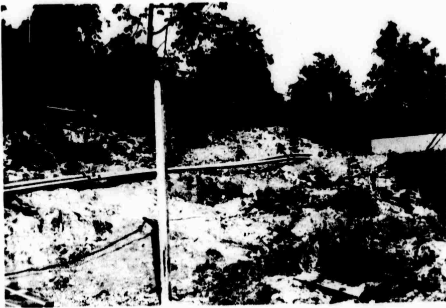
Plate 9: External routing of cables through 4" PVC pipe. AC power pole is in center; WWSSN vault and recording building is on the right.
