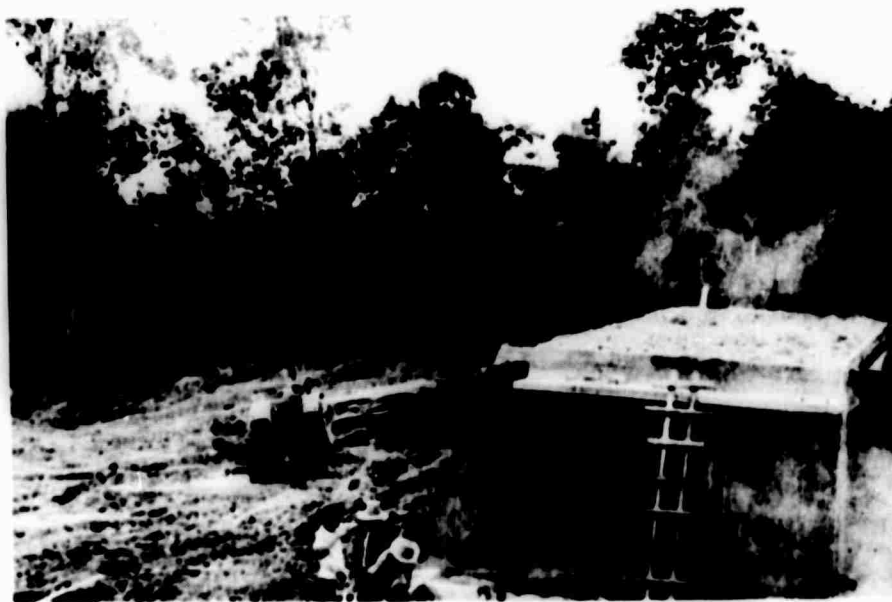
Plate 4: Backfilling around the vault.
