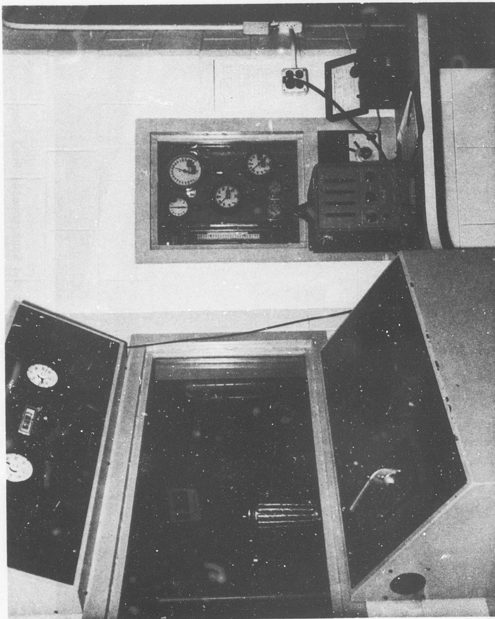
Figure 12. Laboratory Control Room and Pump Instrumentation.
